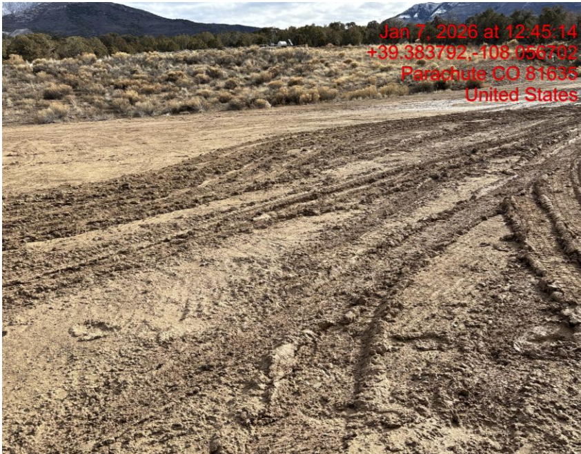
Lack of Stabilization – Photo #02238
