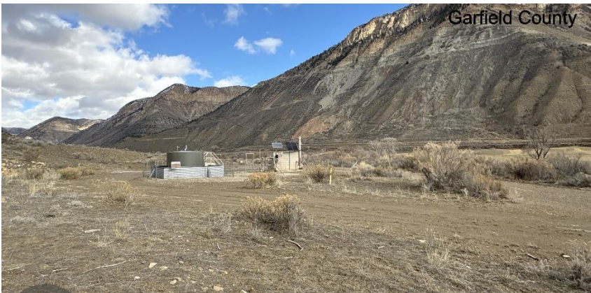
South West corner of location.
