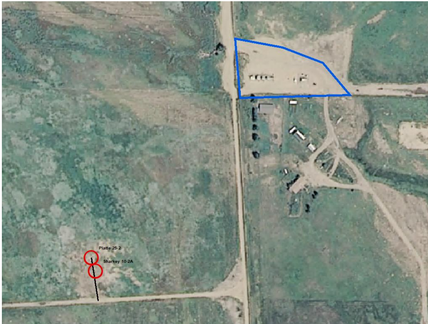
Photo 1. NAIP aerial imagery (2009) illustrating the well locations (red circles), associated tank battery location (blue polygon), and well and TB access road (black line). The tank battery is associated with the Helen Marie Purse B1 well API #123-08001 under location ID #317939.
