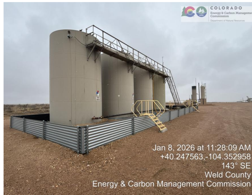
Photo 4 tank battery and production equipment
