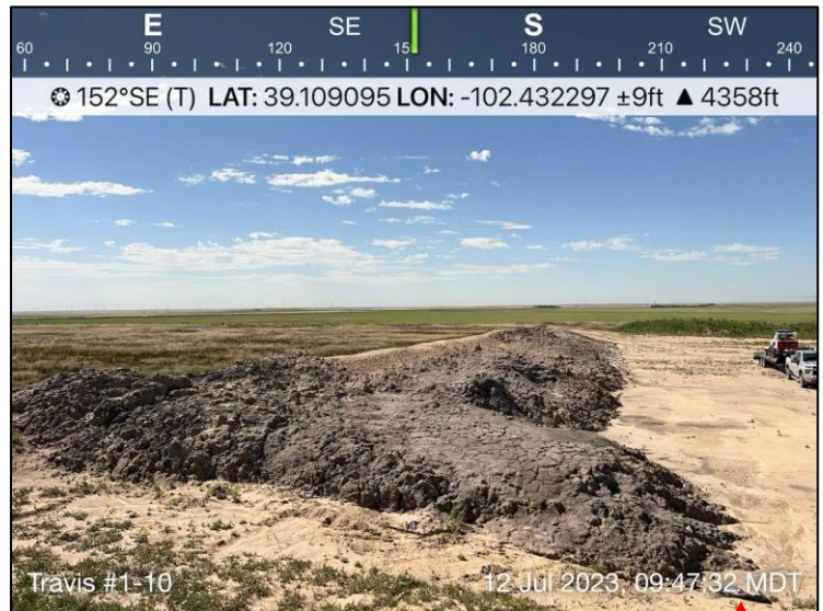
Figure 3. Demonstrates dried drill cuttings still on liner (7/12/23)
