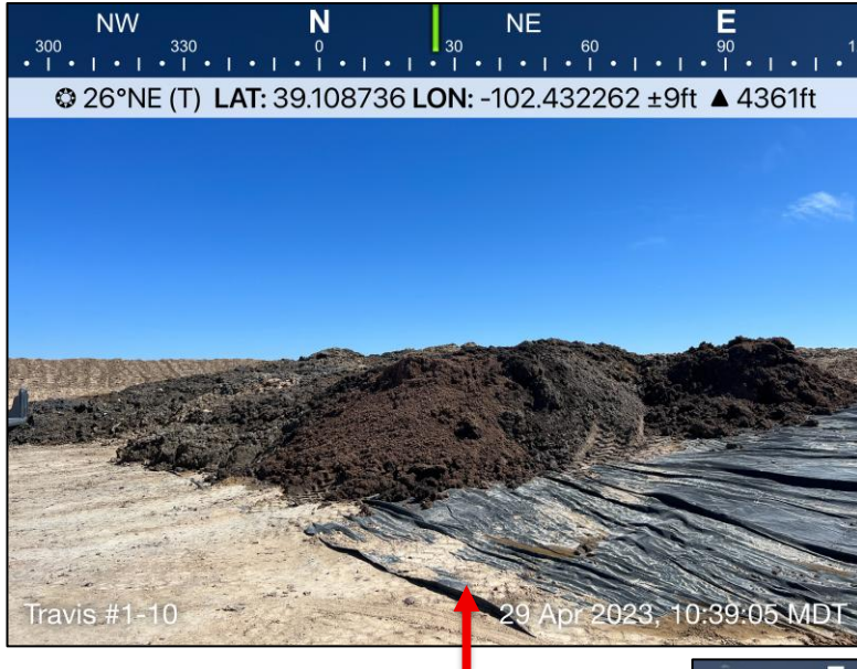
Figure 2. Demonstrates dried drill cuttings on liner (4/29/23)
