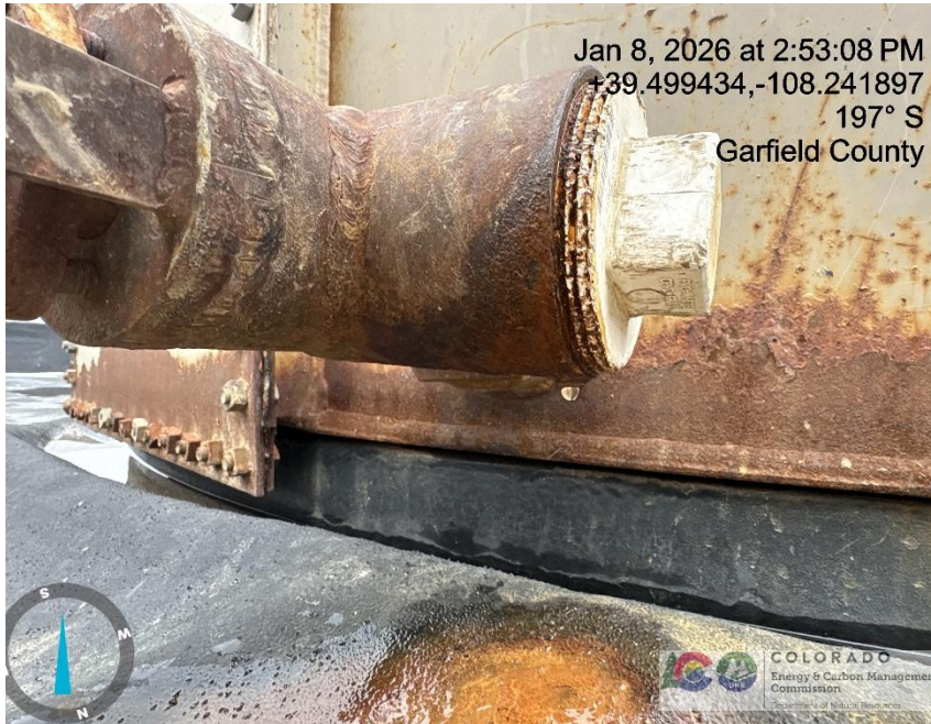
Photo # 9661 Mechanical Condition - Possible leak on tank valve
