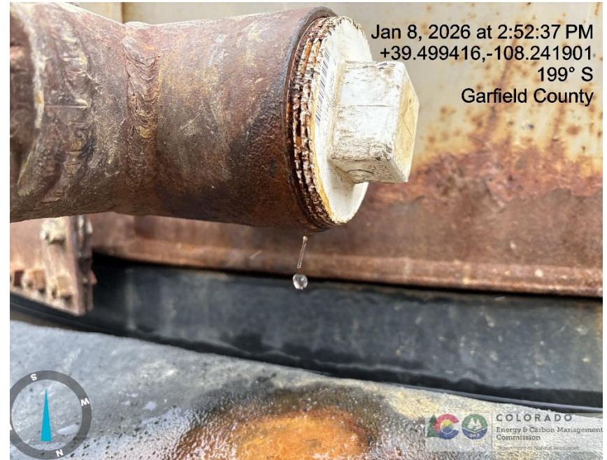
Photo # 9662 Mechanical Condition - Possible leak on tank valve
