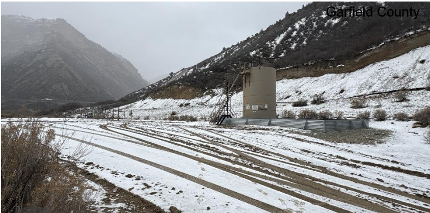
South West corner of location.
