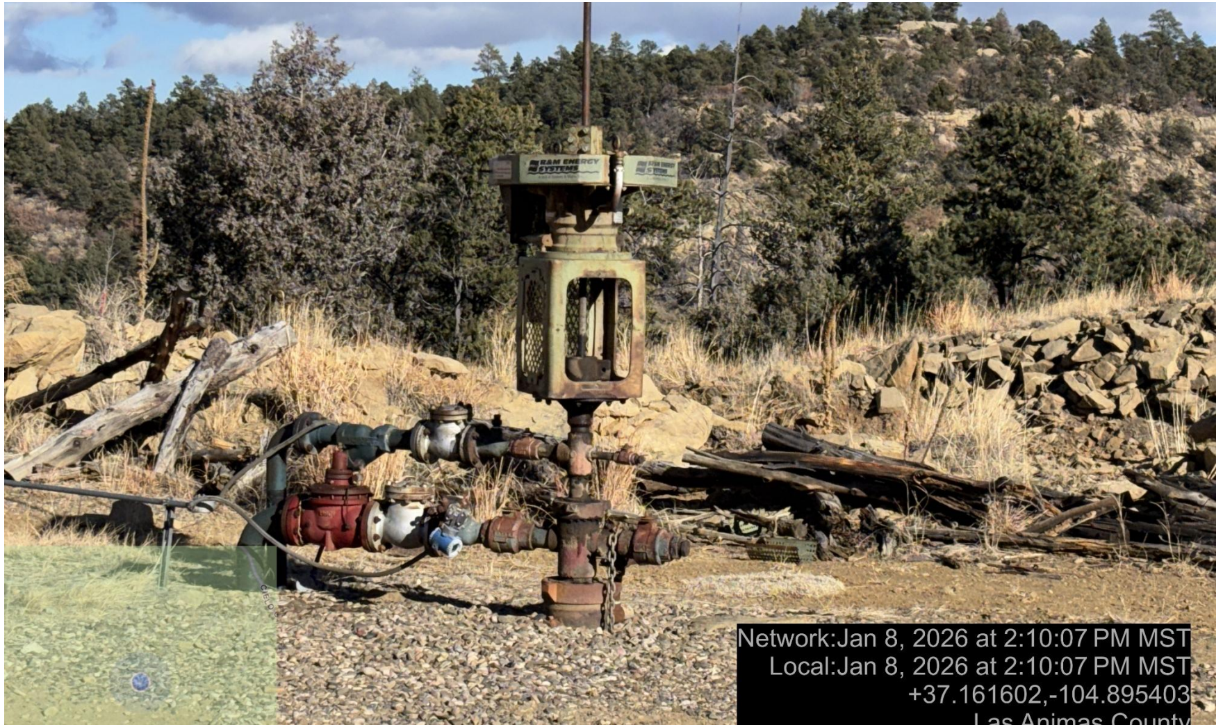
PHOTO 4: ORIGINAL WELLHEAD AND EQUIPMENT.
