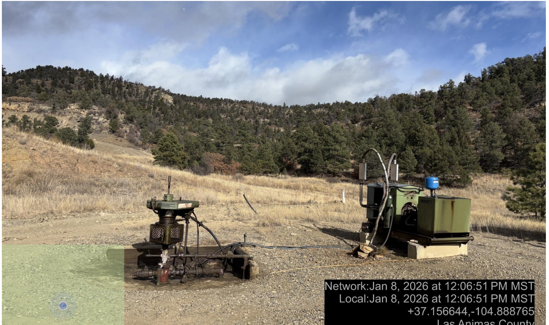
PHOTO 4: WELLHEAD AND EQUIPMENT.
