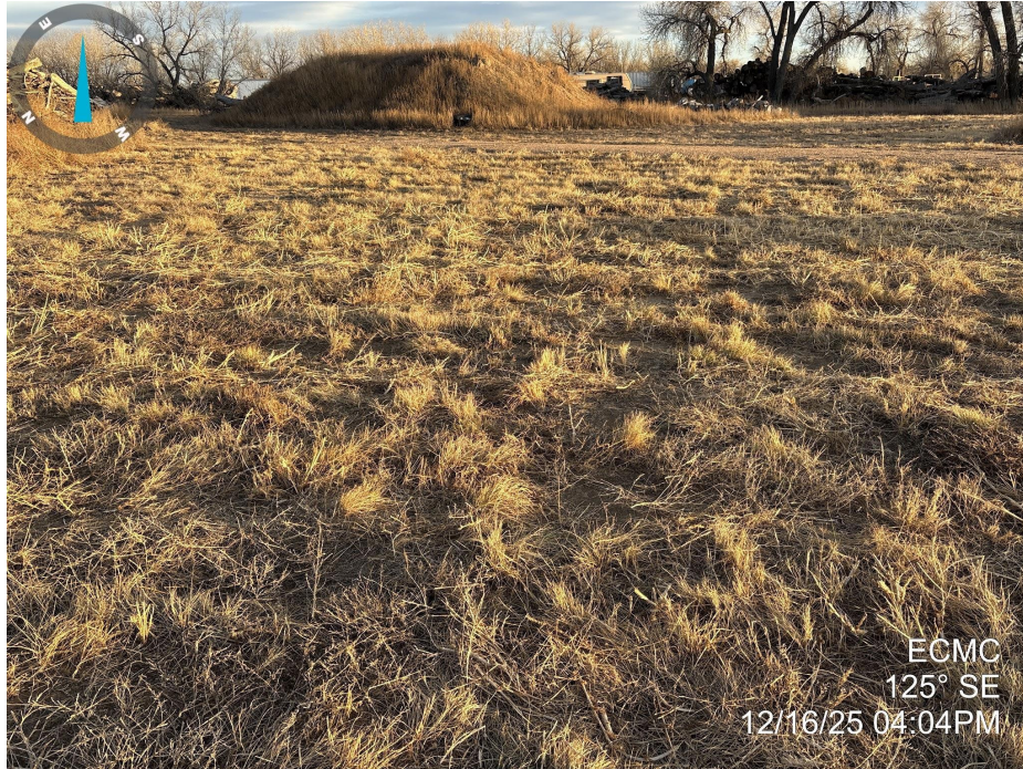
Photo 5. Photo taken of the tank battery location, facing southeast. Photo illustrates that final reclamation activities appear to have taken place. However, the location has been recently mowed, so vegetation establishment will be determined in a future inspection.
