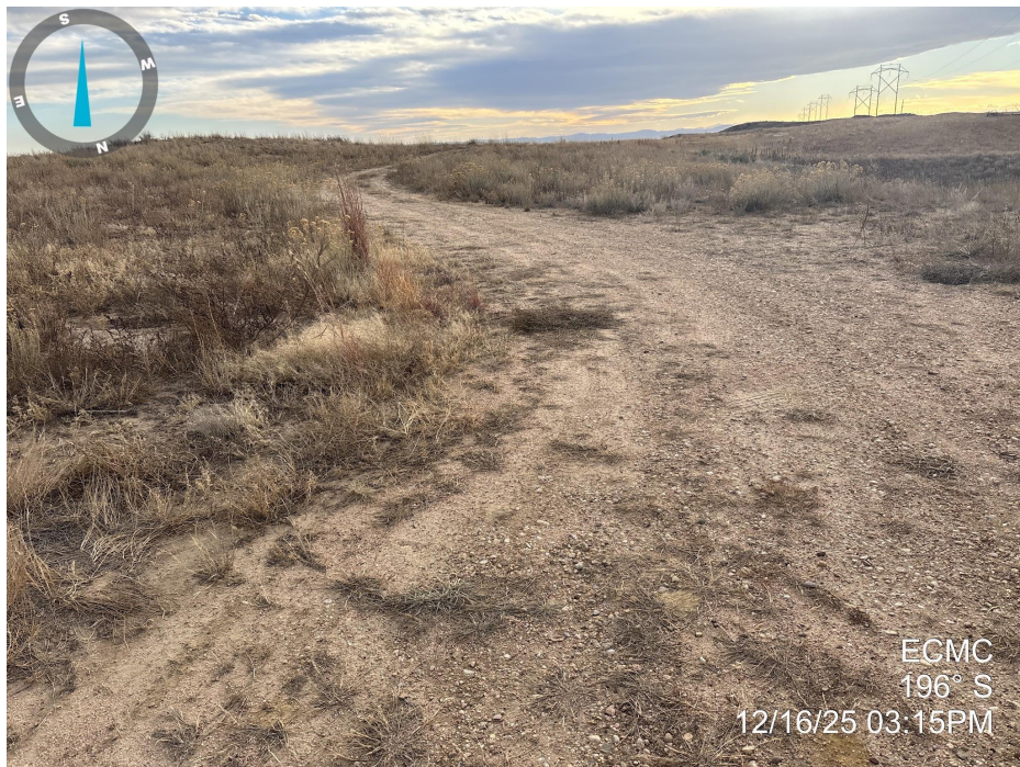
Photo 5. Photo taken of the access road to the location, facing south, towards the location. Photo illustrates that final reclamation activities have not taken place and gravel and bare ground remain across the road.
