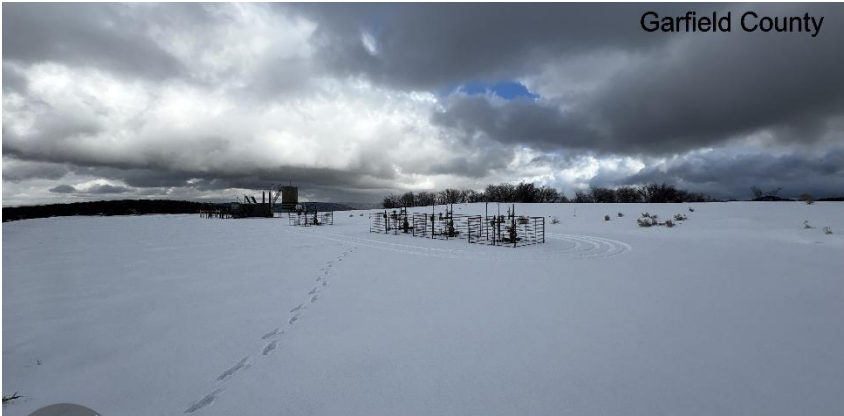
South West corner of location.
