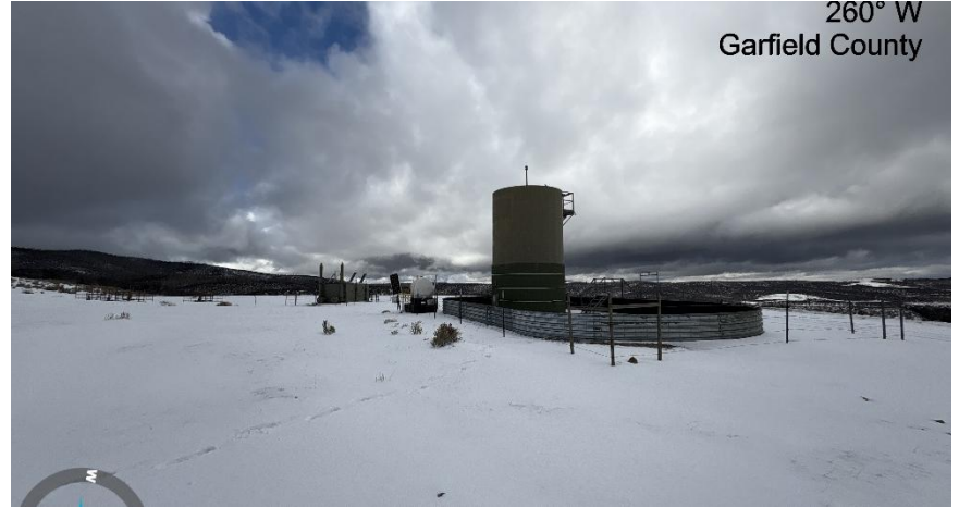
North East corner of location.
