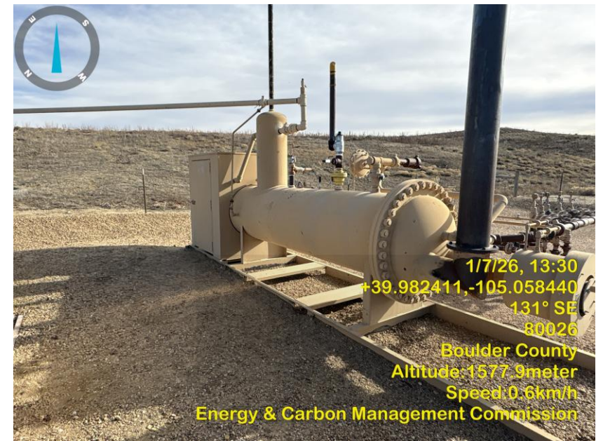
Photo 4 Horizontal Heated Separator.
