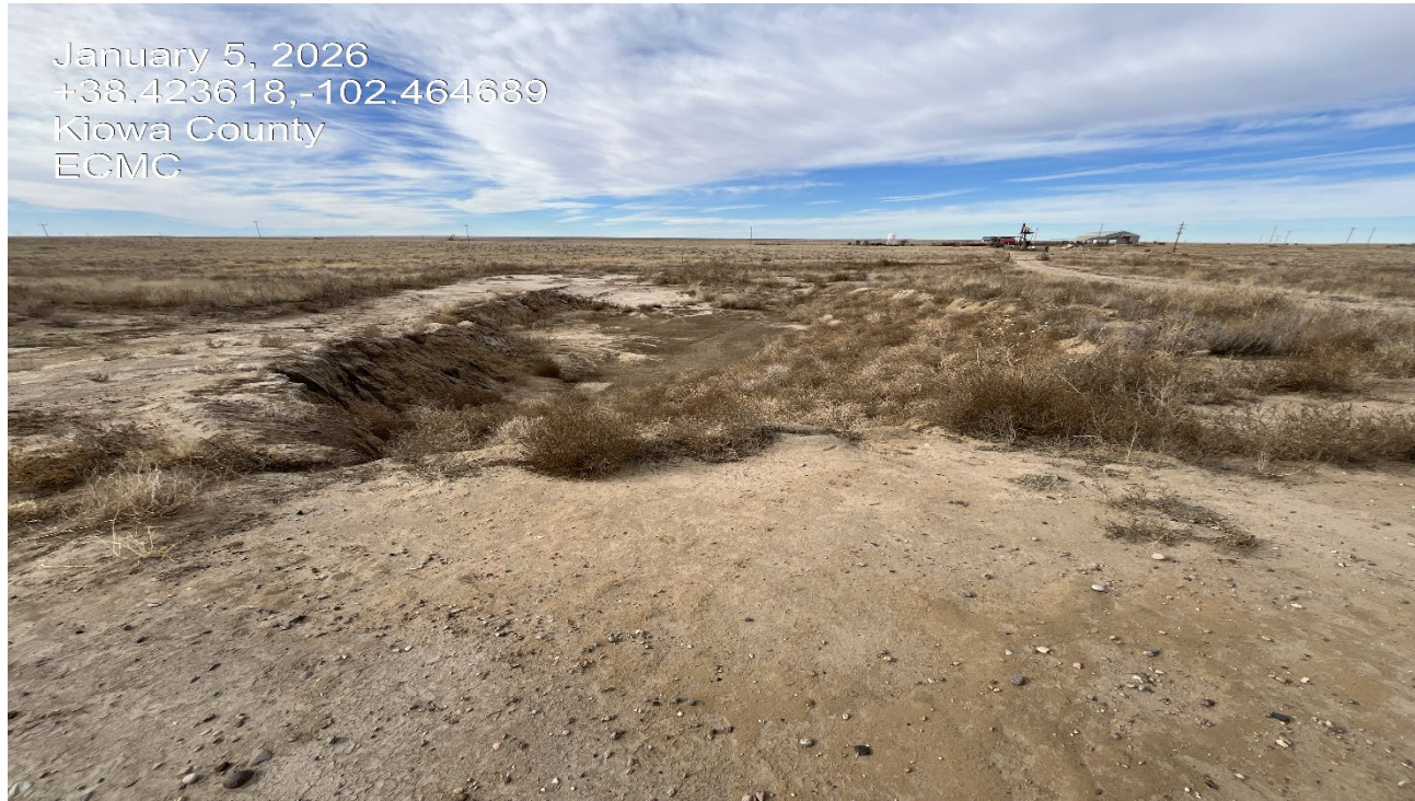
Photo 3. Facing east toward the remediation excavation area. Remediation remains in process and has been ongoing since 2022. There is undesirable weed debris accumulated inside the excavation.
