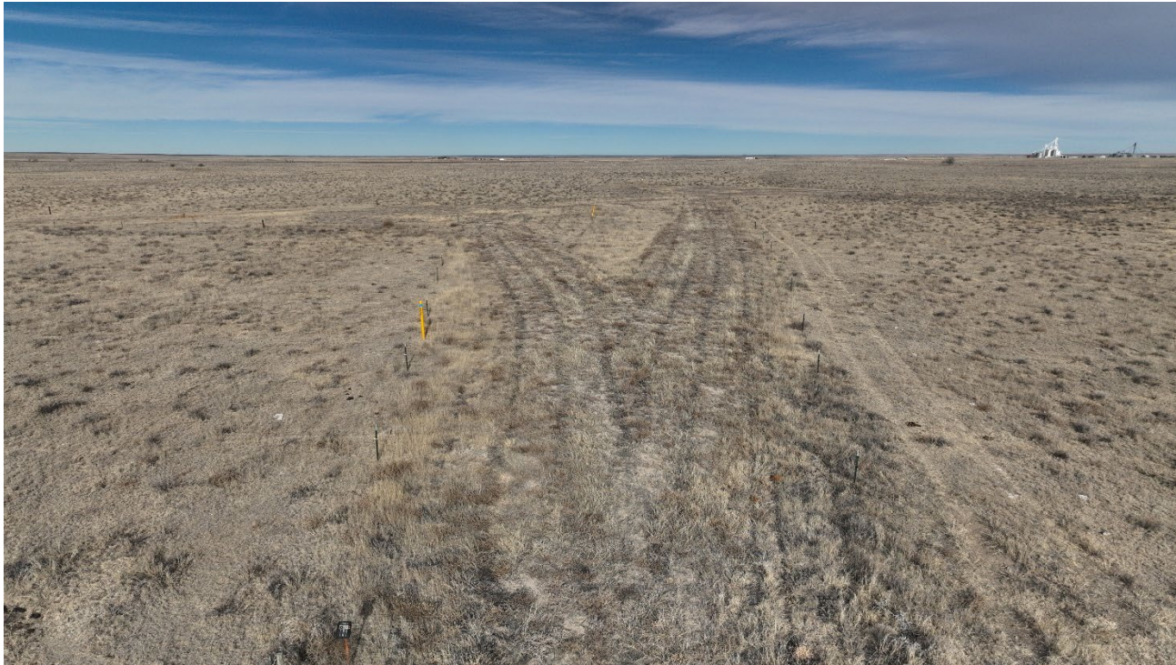
Photo 3. Drone aerial photo facing north overlooking the reclaimed portion of the road and location.
