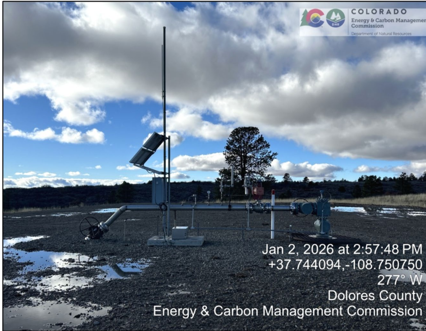
03. Kinder Morgan DC #6 well head assembly and meter run.
