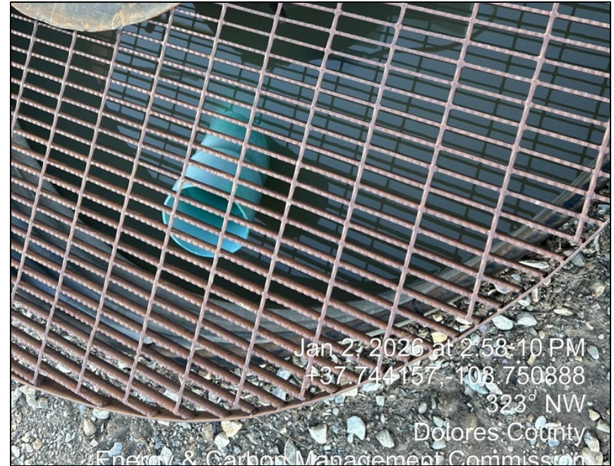
06. DC #6 well cellar. Cellar is half full of water. Bradenhead access appears to be inside of PVC pipe.
