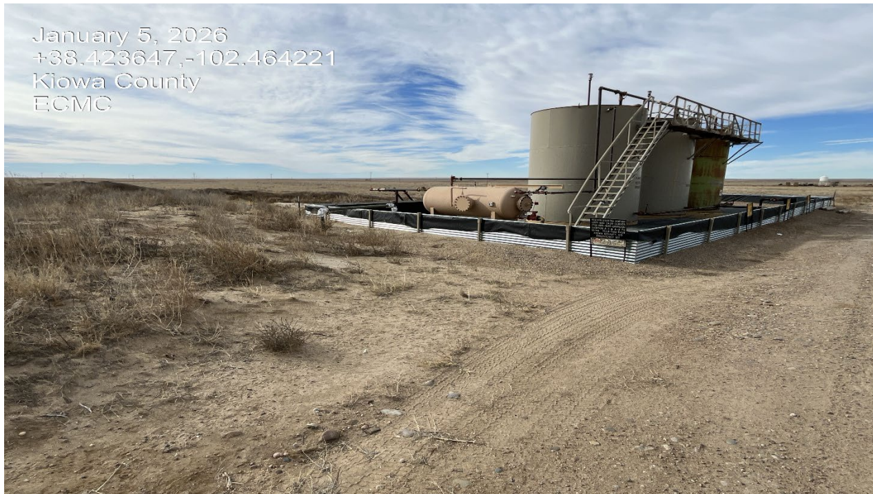
Photo 1. Facing southwest toward the Dawson A 1 tank battery.
