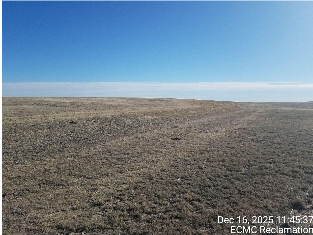
Photo 3. Photo taken from a portion along the eastern access road and west of the location, facing East. Photo illustrates the Operator has performed additional final reclamation activities by importing new topsoil, and reseeded the location with the evidence of straw crimped mulch.
