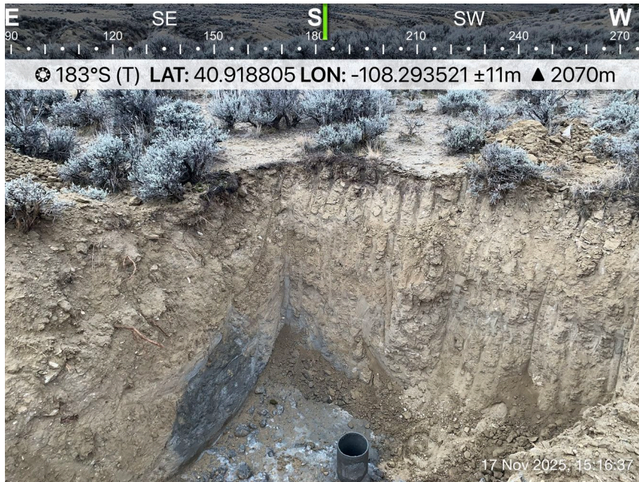
Photo 4: State #31-16 (OWP) P&A well, view south, no methane detected.
