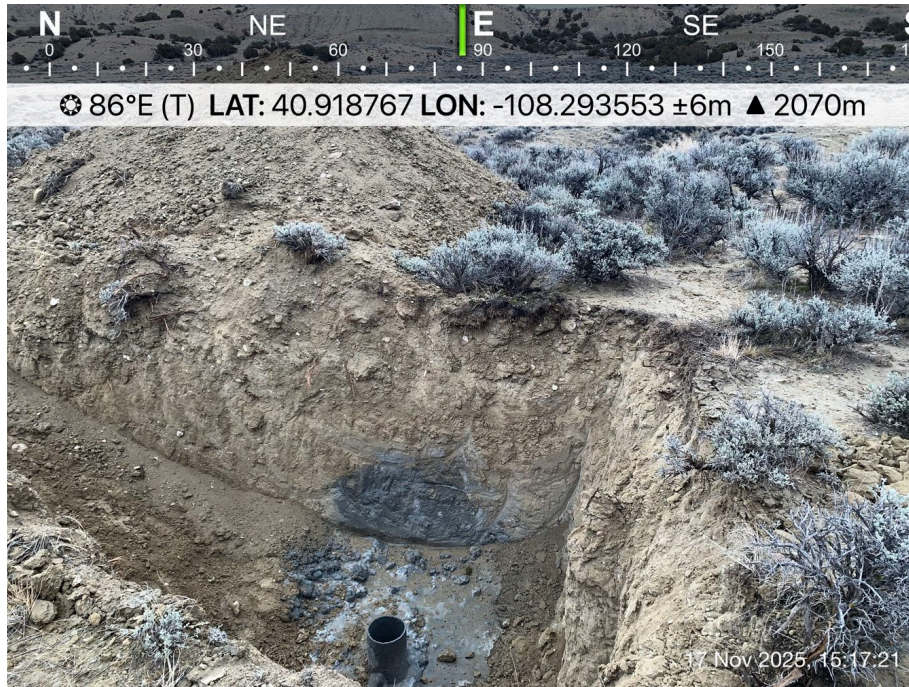
Photo 3: State #31-16 (OWP) P&A well, view east, no methane detected.
