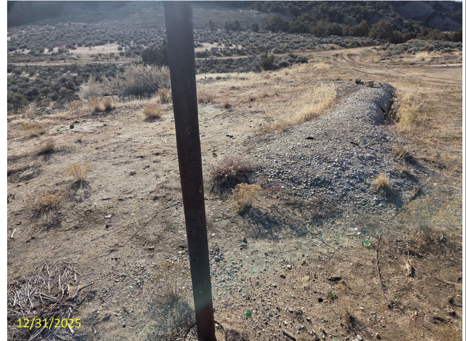
Photo 1: Photos taken from the well site. Photo shows concrete pad/pump base has not been removed and properly disposed.
