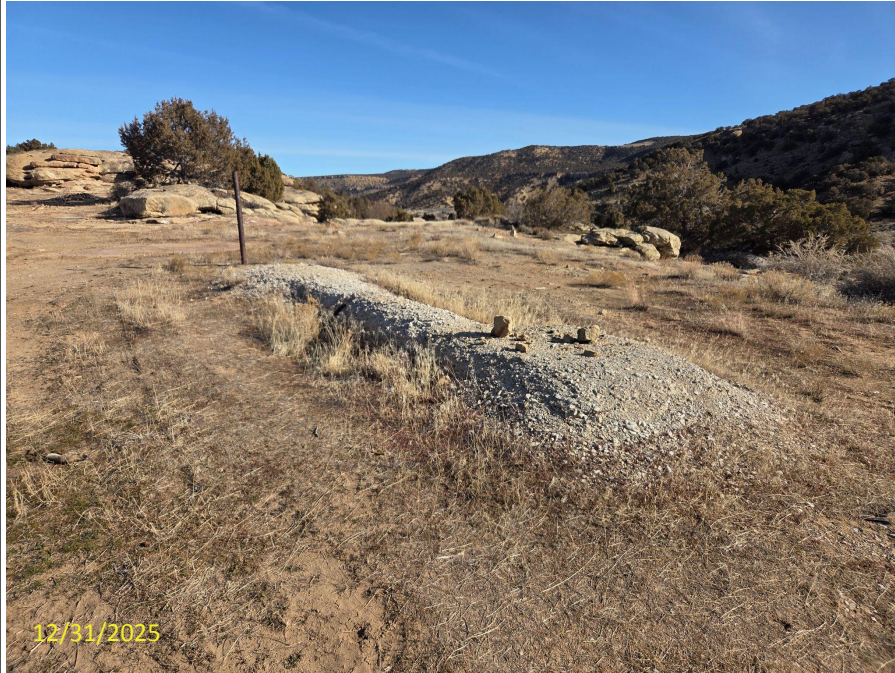
Photo 1: Photos taken from the well site. Photo shows concrete pad/pump base has not been removed and properly disposed.
