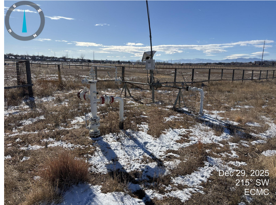
Photo 4. Picture taken at the west side of the tank battery location. Pipe riser and meter remain on location.
