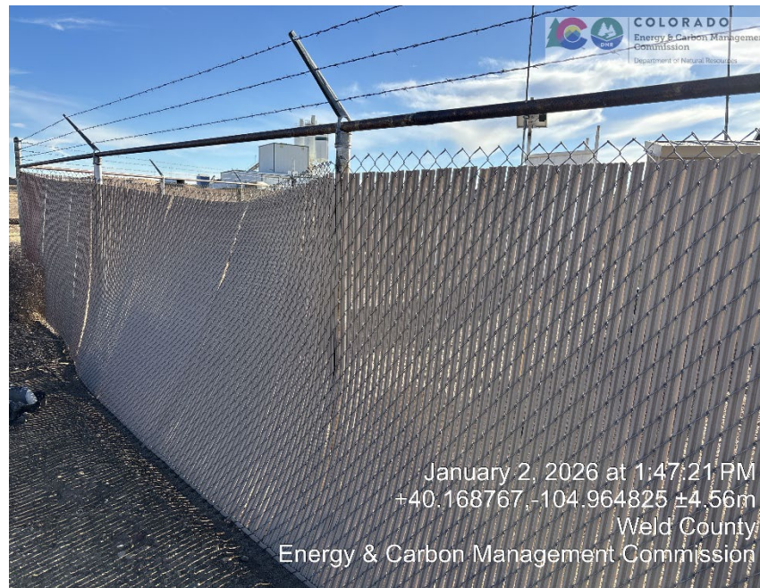
North-east separator fencing
