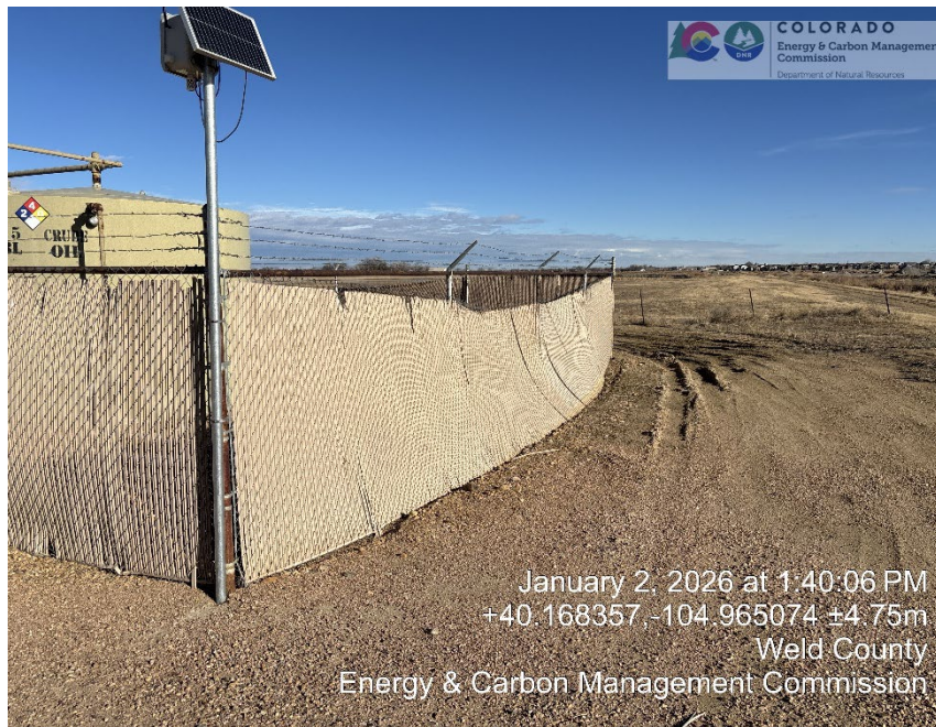
South crude oil tank fencing
