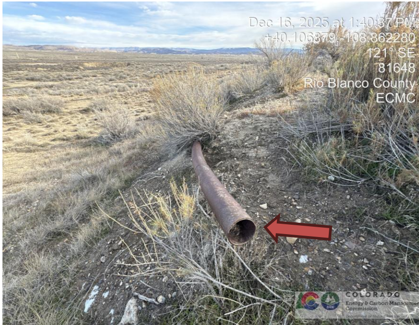
Photo # 0310 Debris on NE side of location
