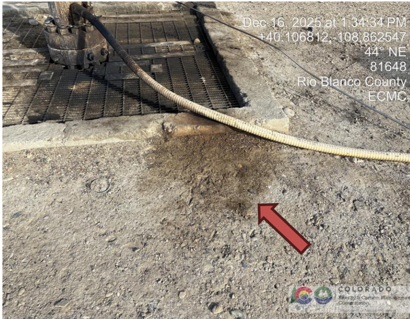
Photo # 0300 Staining on location
