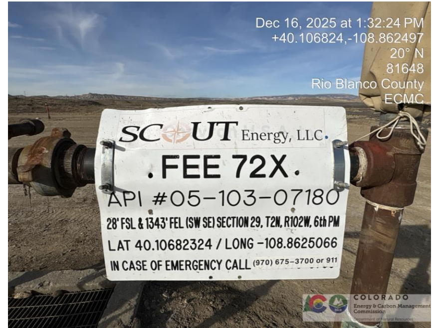
Photo # 0297 Wellhead sign lacks public road used to access the well
