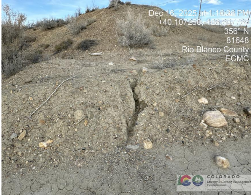
Photo # 0281 Loss of berm integrity due to erosion on north side of location/insufficient BMP's
