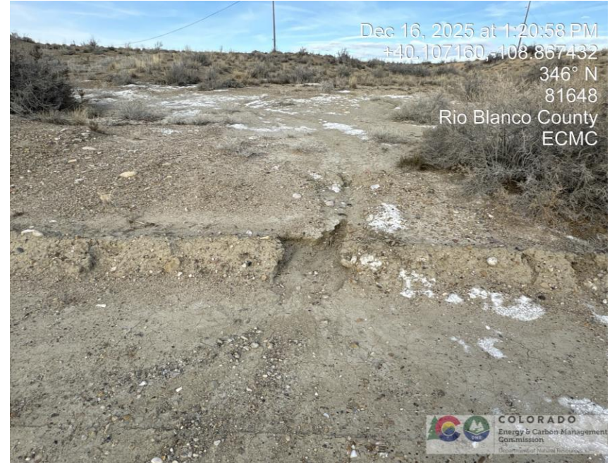
Photo # 0286 Loss of berm integrity due to erosion on north side of location/insufficient BMP's
