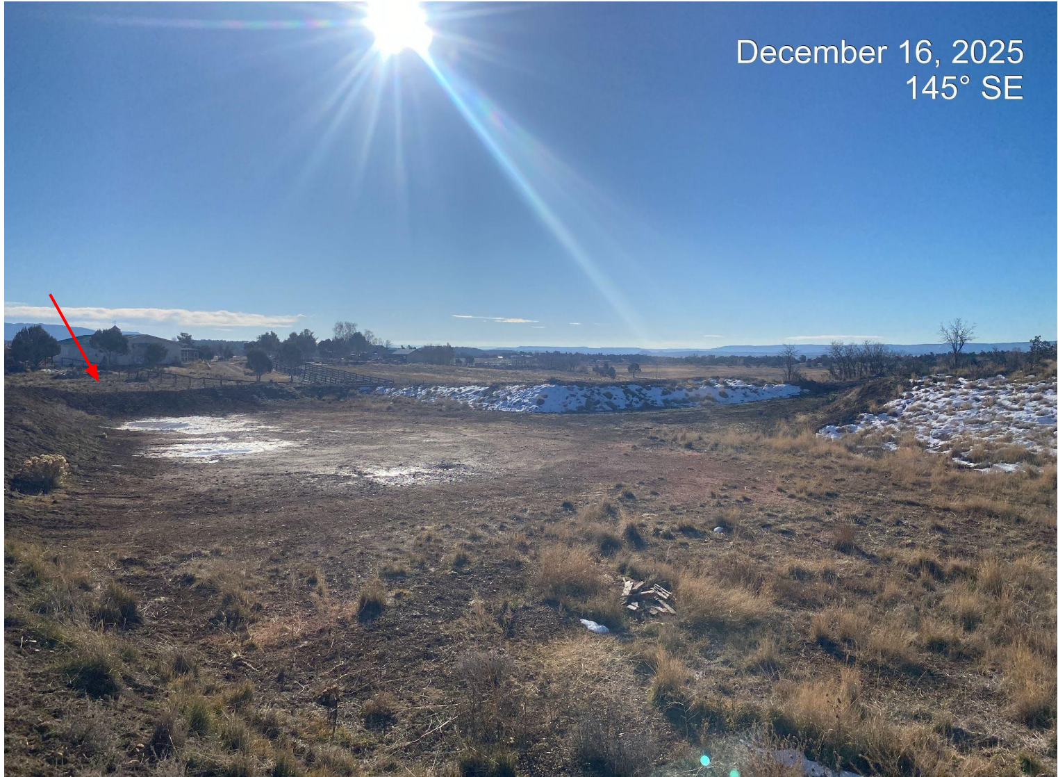
Photo 3. View of the the western portion of the project area taken from the northern edge facing south east. Note: Additional berm has been constructed on the southern edge of the western project area (indicated by red arrow). It was noted that surface owner equipment has been removed but western portion of the project area still remains unreclaimed per 1004 rules.
