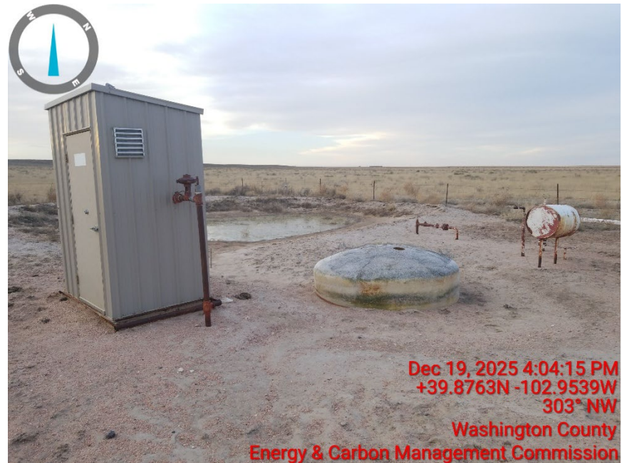
3. East side of VGS shed and buried tank
