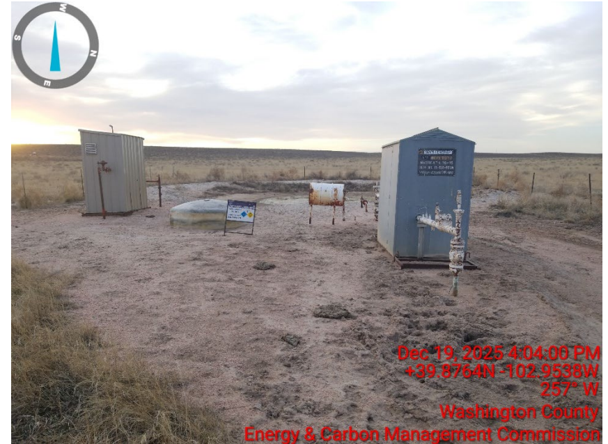
2. Meter shed, VGS shed and fiberglass tank. Lease sign on meter shed has not been updated
