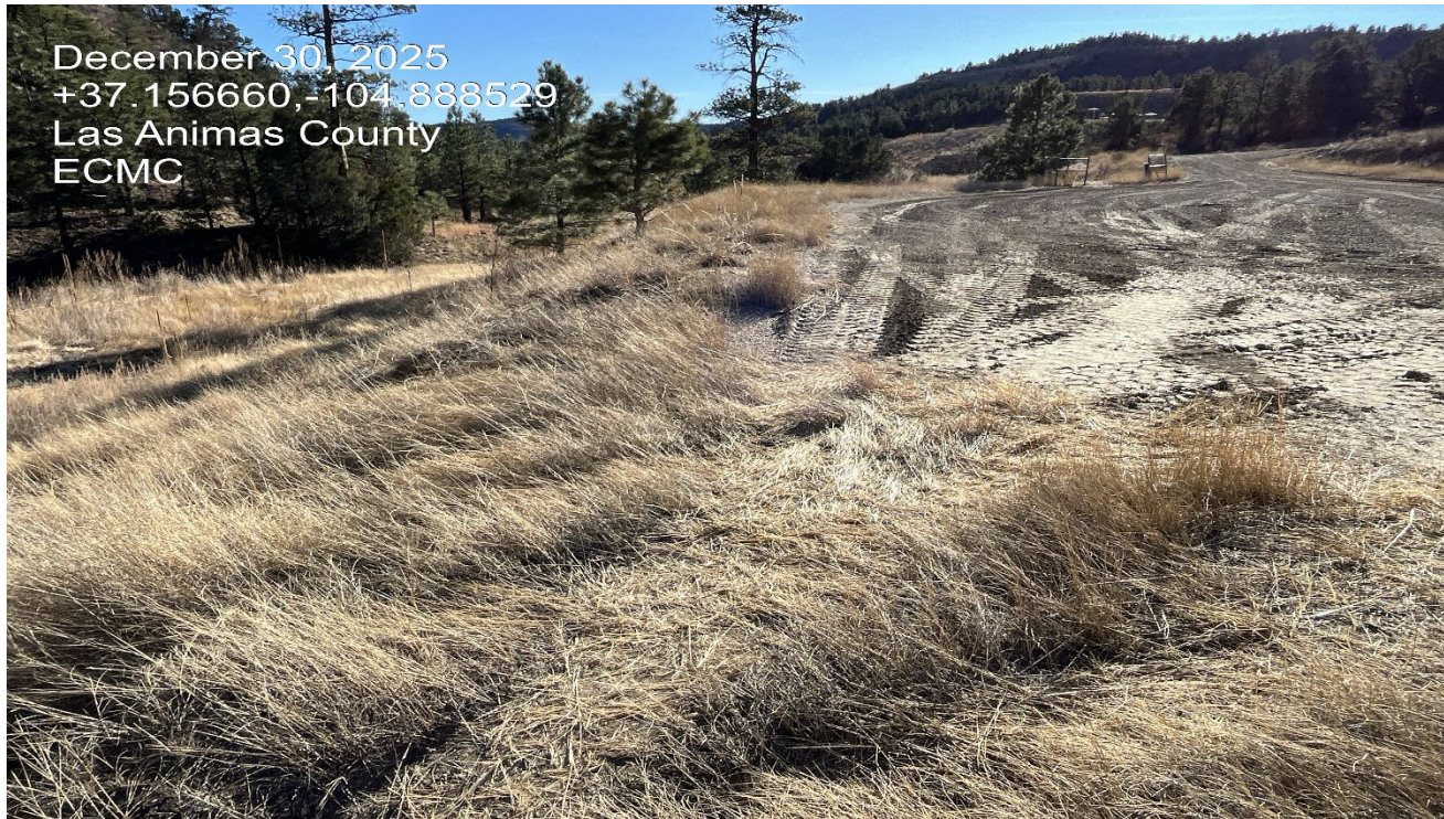
Photo 4. Facing south along the fill slope.
