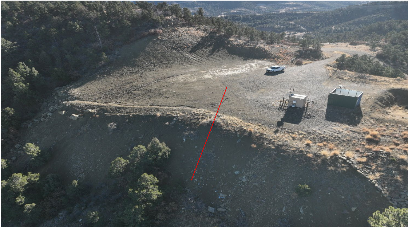
Photo 6. Drone aerial photo facing south. The fill slope material shown approximately to the left side of the line will need to be replaced back into the cut slope.
