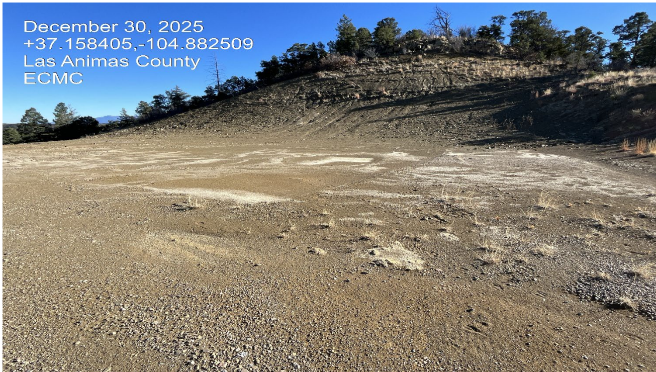
Photo 1. Facing southeast at the PA'd wellsite. The pit has been backfilled and equipment is removed.
