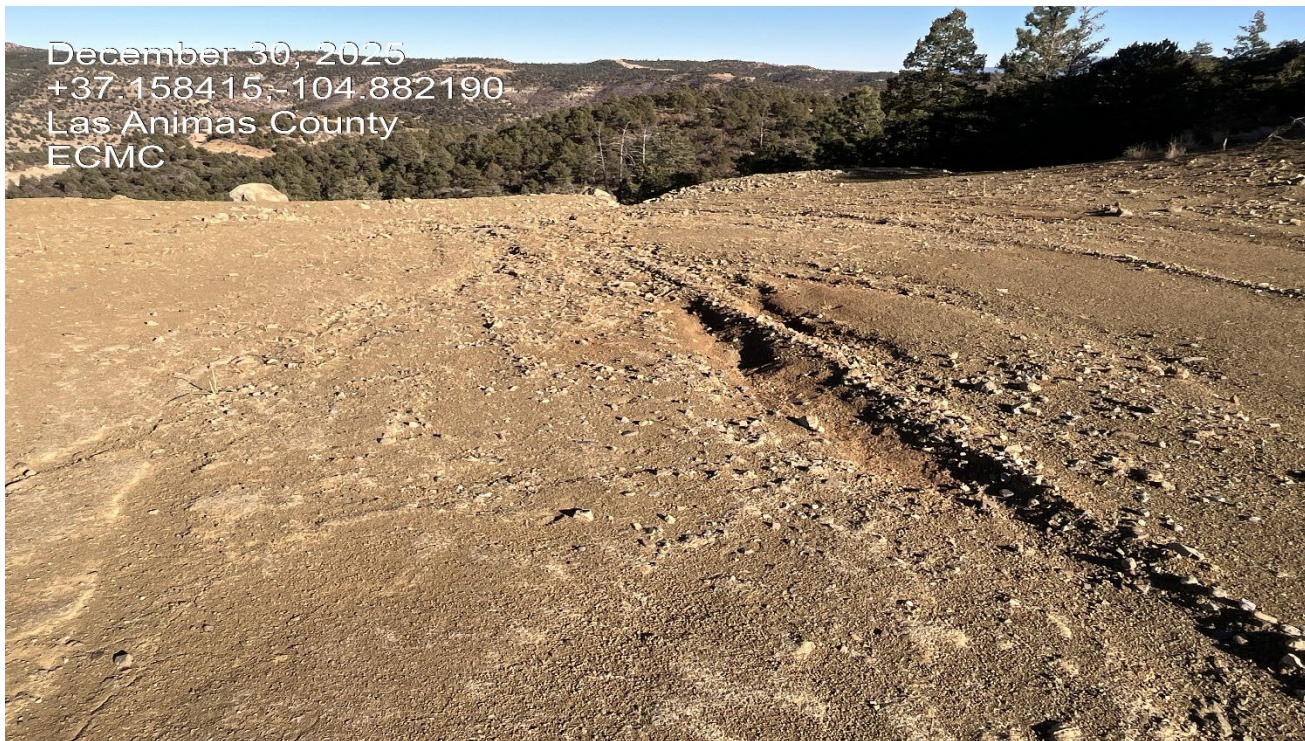
Photo 2. Facing toward the northeast side of the location. There are signs of erosion along this area of the location and soils are not stabilized.
