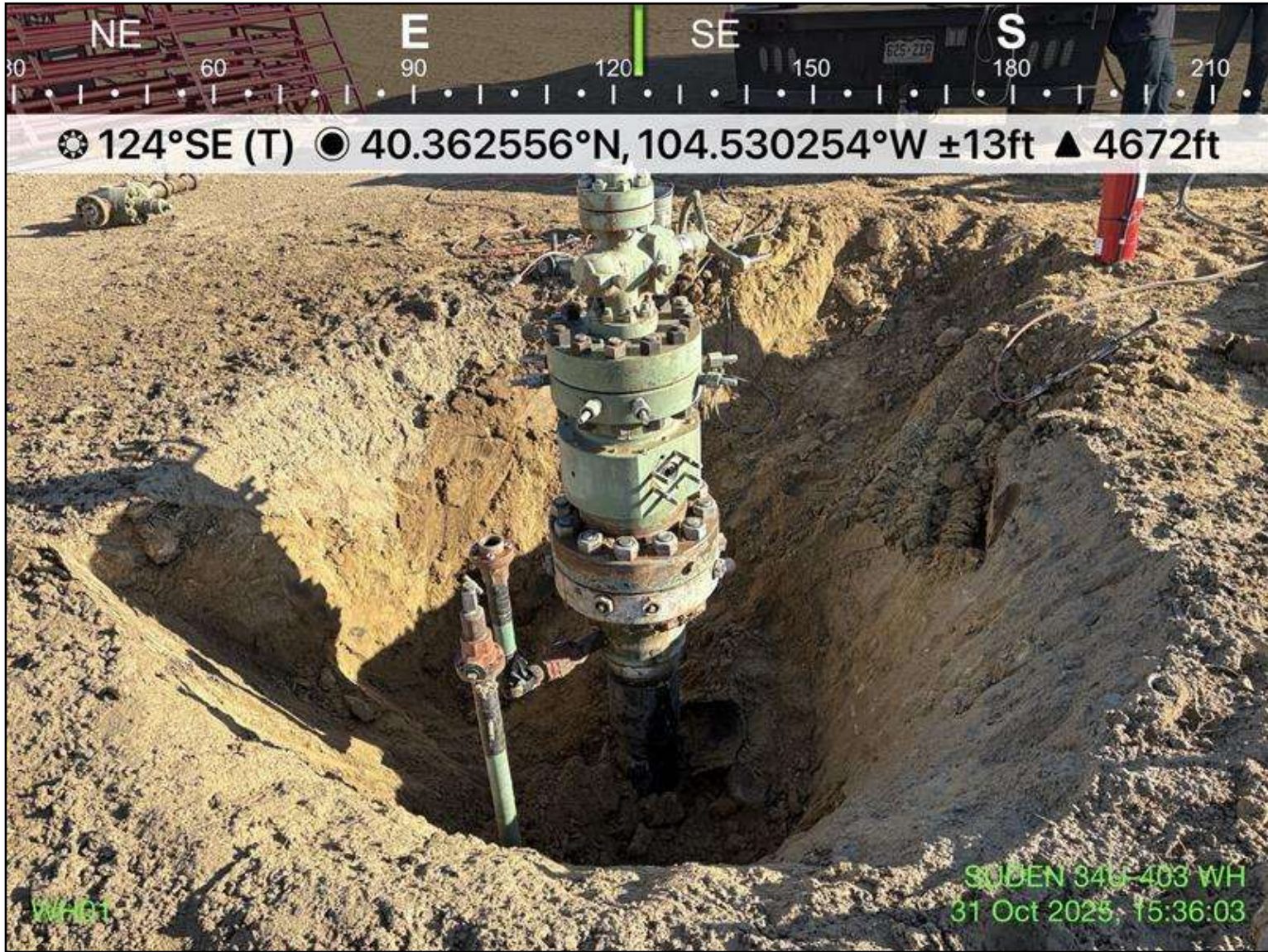
Photo 2: View of wellhead excavation, facing southeast
