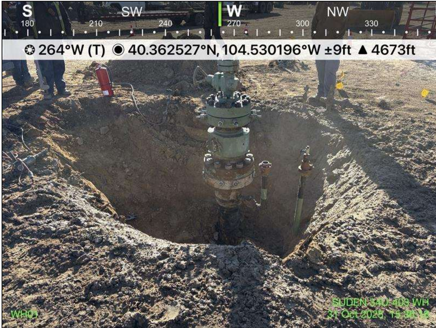
Photo 6: View of wellhead excavation, facing west
