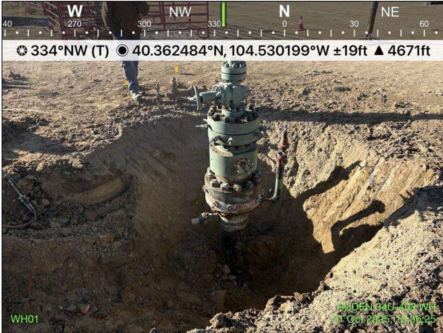
Photo 4: View of wellhead excavation, facing northwest
