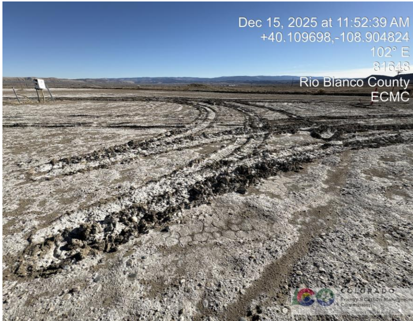
Photo # 0206 Lack of stabilization/Compaction on location
