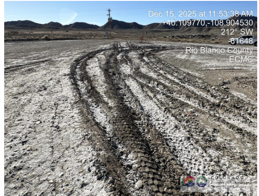
Photo # 0209 Lack of stabilization/Compaction on location
