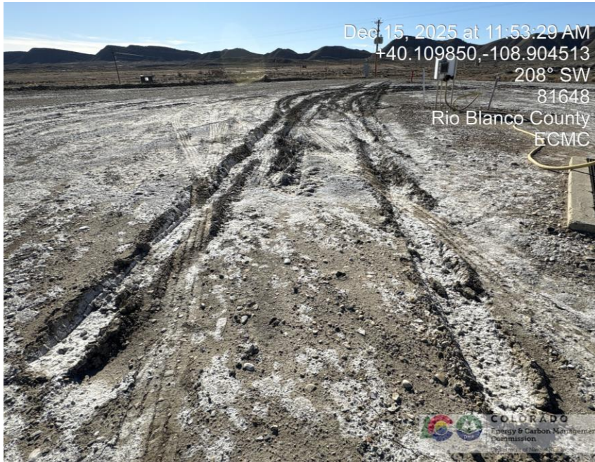
Photo # 0208 Lack of stabilization/Compaction on location
