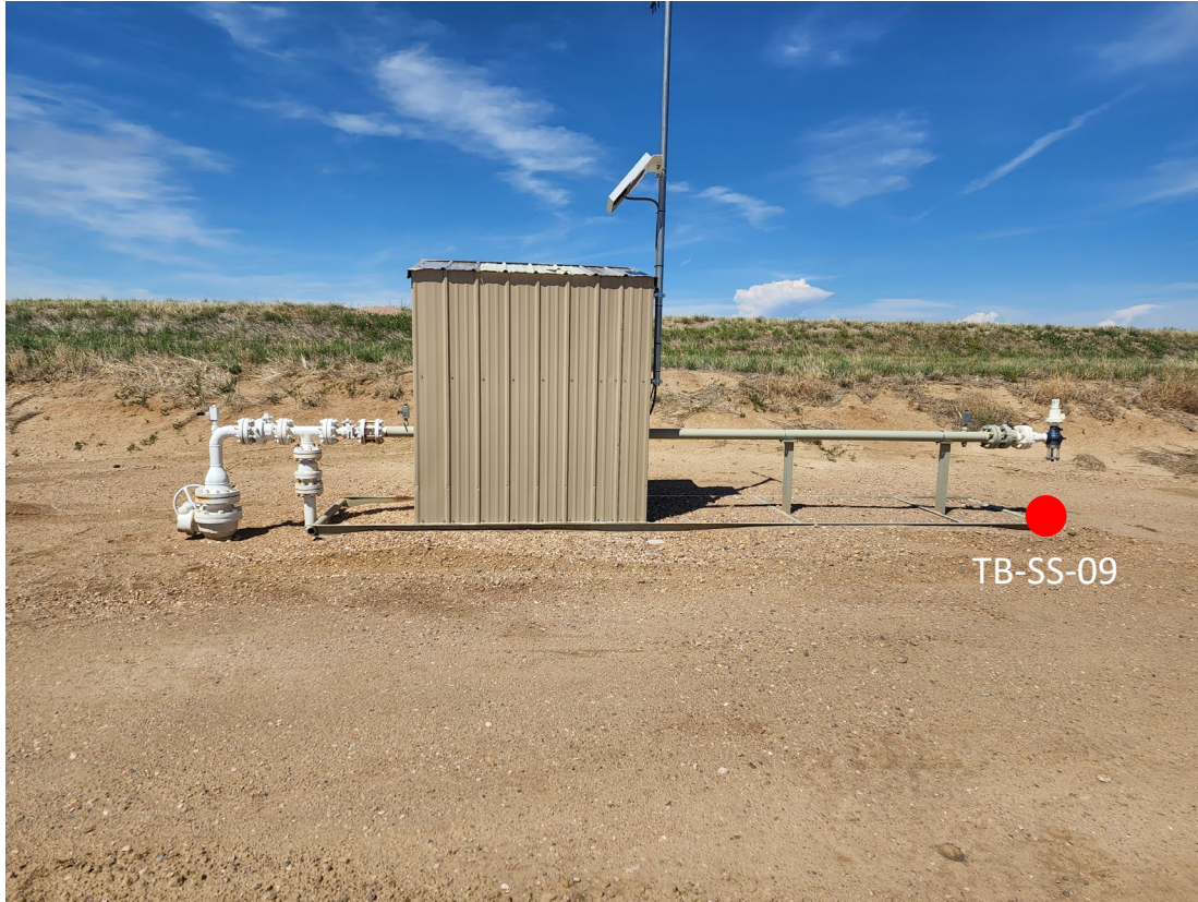
Looking west at meter house
