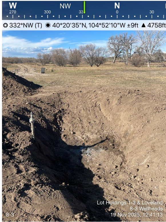
Loveland 8-3 Wellhead Excavation
