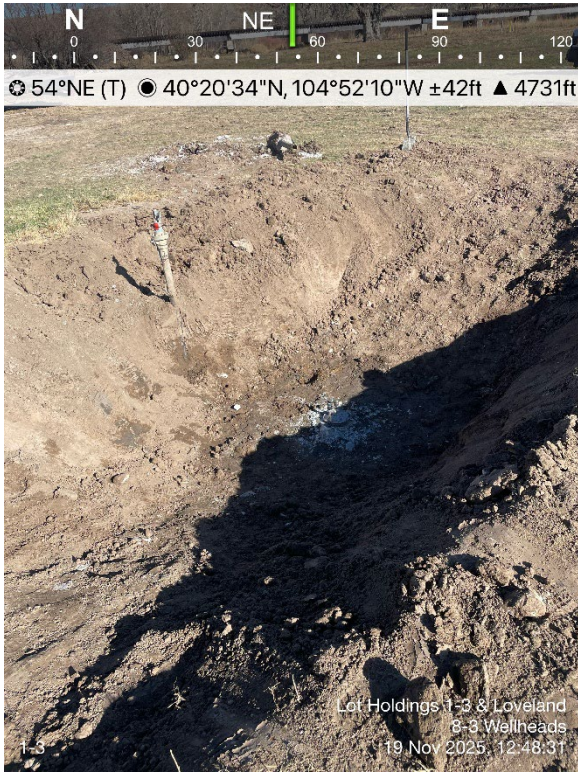
Lot Holdings 1-3 Wellhead Excavation
