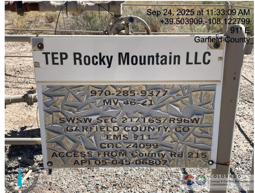
Photo # 2174 From inspection/audit 708907542 conducted on 09/24/2025 - Illegible Wellhead Sign
