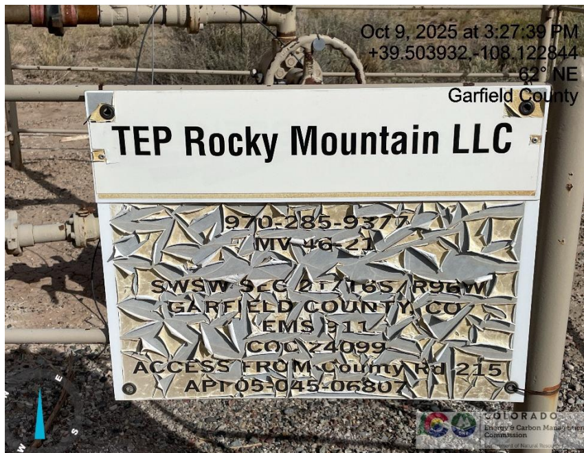
Photo # 5811 From inspection/audit 708907638 conducted on 10/09/2025 - Illegible Wellhead Sign
