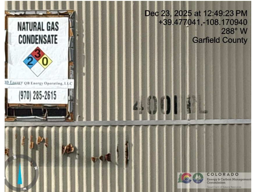
Photo # 5629 Capacity on production tank weathered & starting to become illegible
