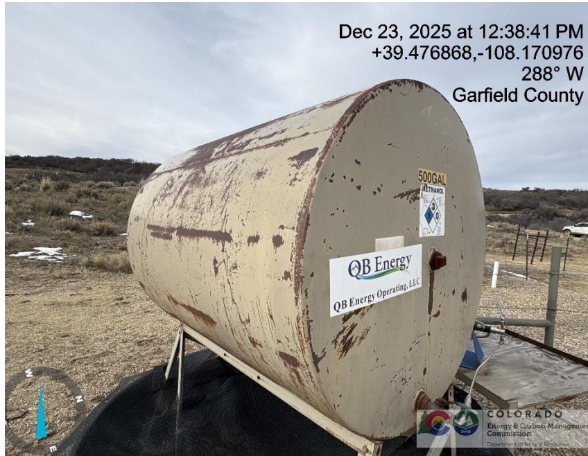
Photo # 5626 Methanol tank lacks required information
