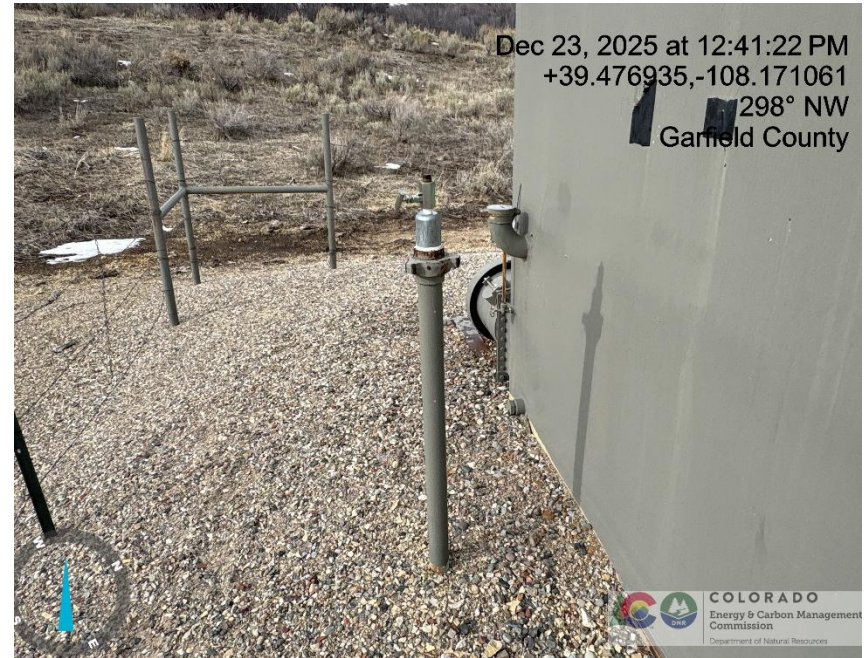
Photo # 5625 Unused flowline lacks lockout tagout (OOSLAT)
