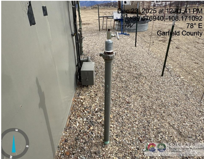
Photo # 5624 Unused flowline lacks lockout tagout (OOSLAT)
