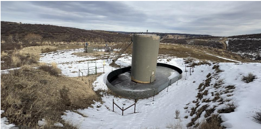
South West corner of location.
