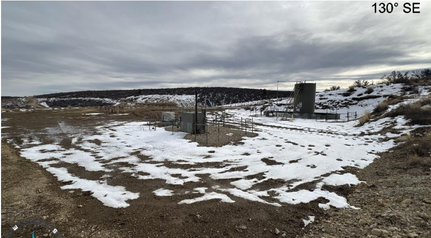
North West corner of location.
