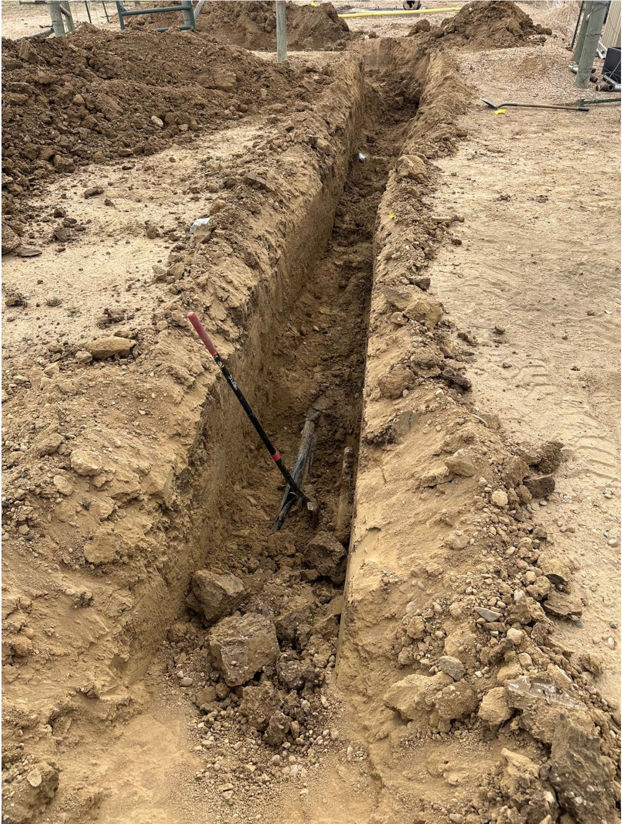
Dumpline Removal Trench
