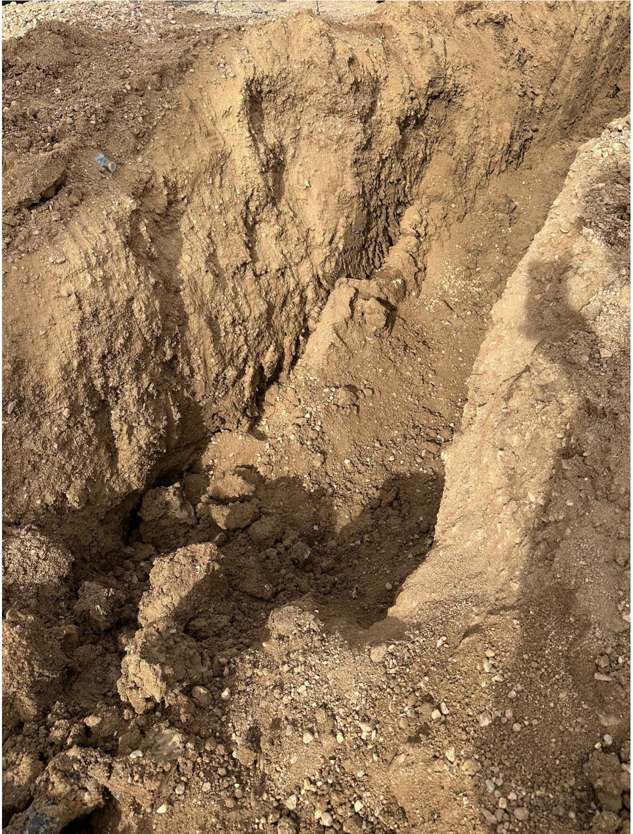
Dumpline Removal Trench
