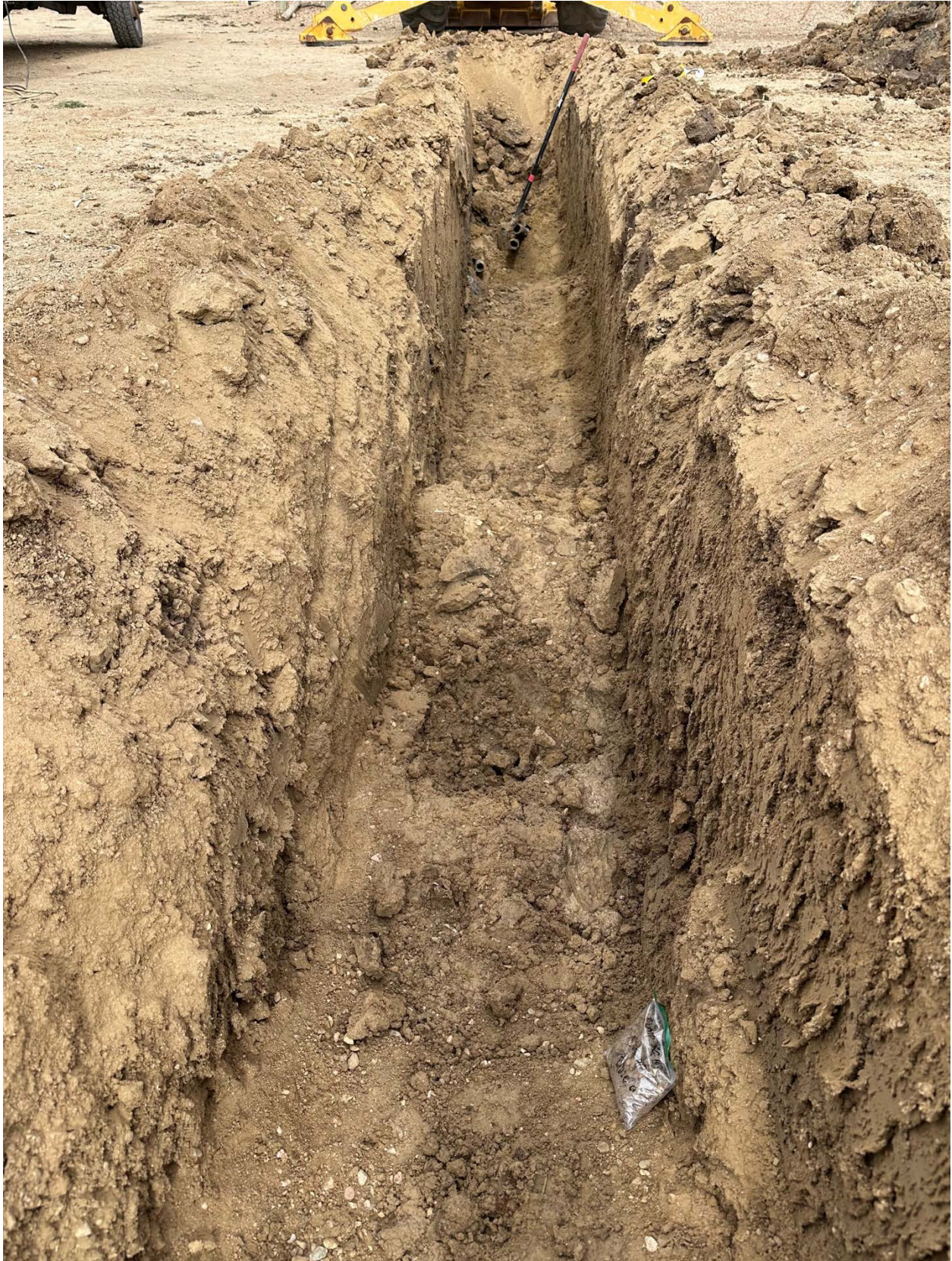
Dumpline Removal Trench - Screening Point: DUMP SCN @ 3' PID: 1.4
