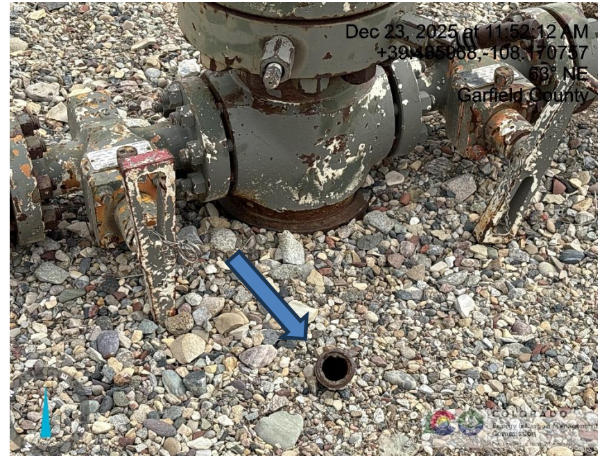
Photo # 5471 Open ended piping near wellhead/wildlife hazard/available for entry by wildlife
