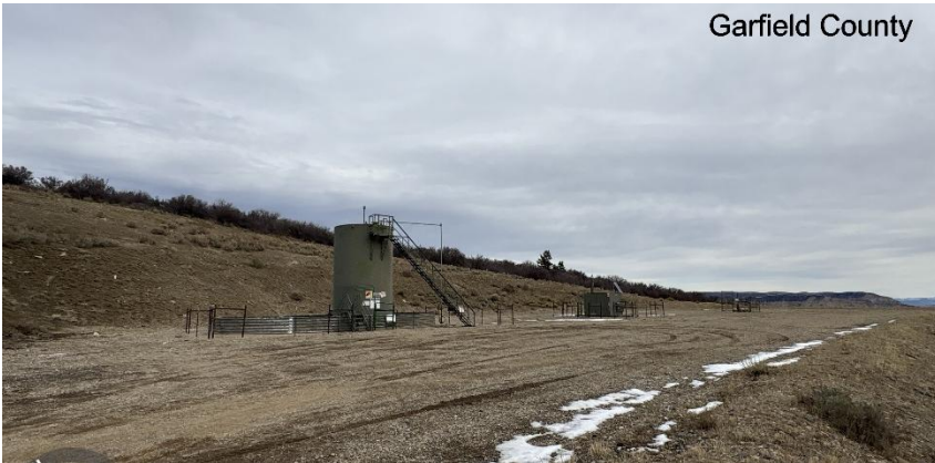
South West corner of location.
