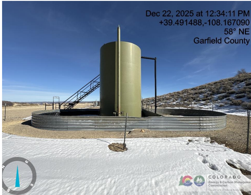
Photo # 4969 Battery lacks required signage
