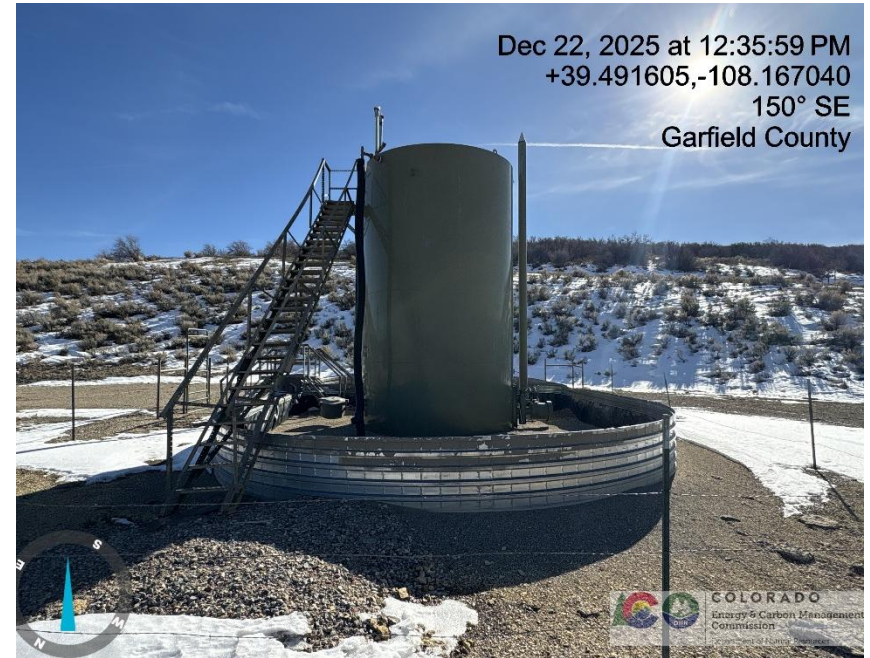
Photo # 4968 Battery lacks required signage
