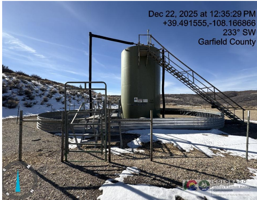
Photo # 4967 Battery lacks required signage
