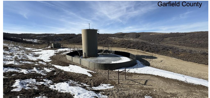
South East corner of location.
