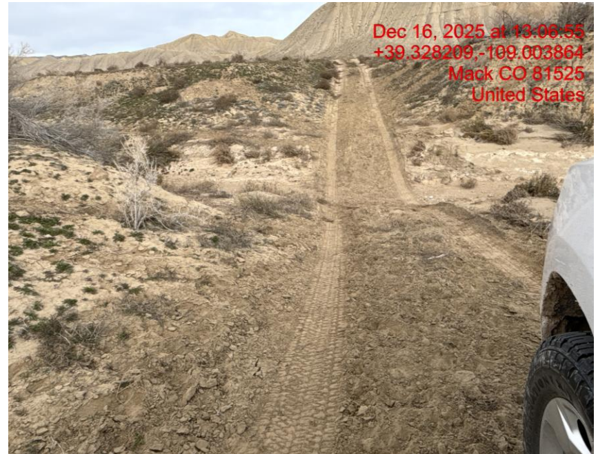
No BMPs Installed at Water Drainage/Stream Crossing – Photo #02036
