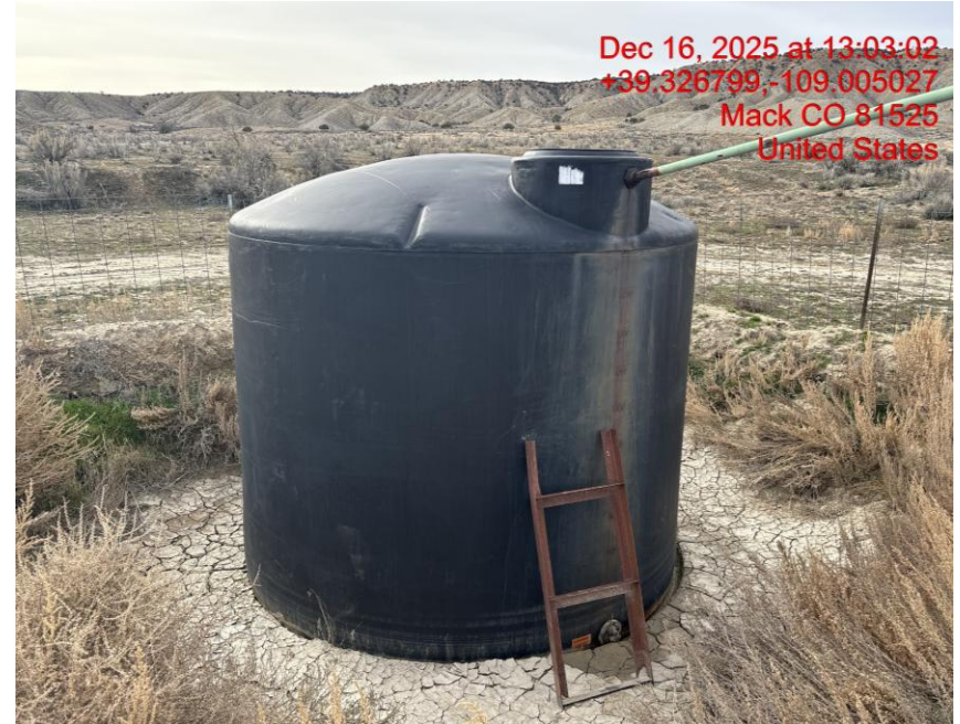
Location/Weeds in Secondary Containment/No Labeling on Tank – Photo #02030
