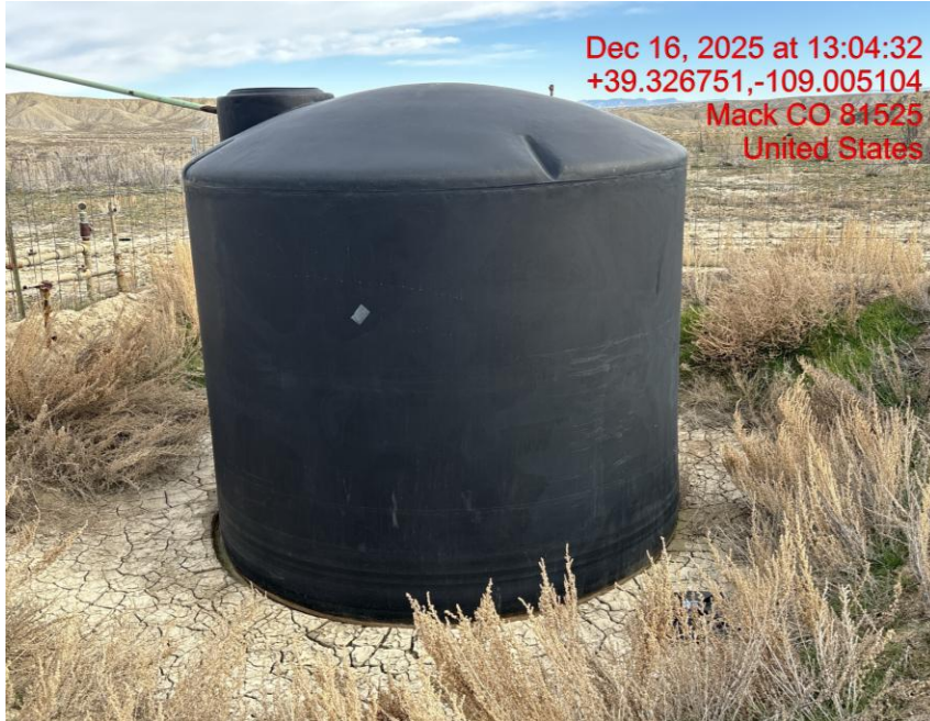
Weeds in Secondary Containment/No Labeling on Tank – Photo #02034
