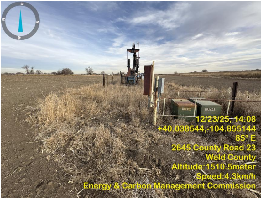
Photo 5 Ancillary equipment overrun with dead vegetation.
