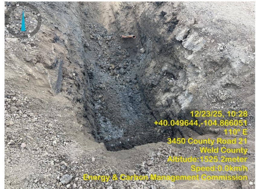
Photo 8 Excavation hole exposing flow lines.
