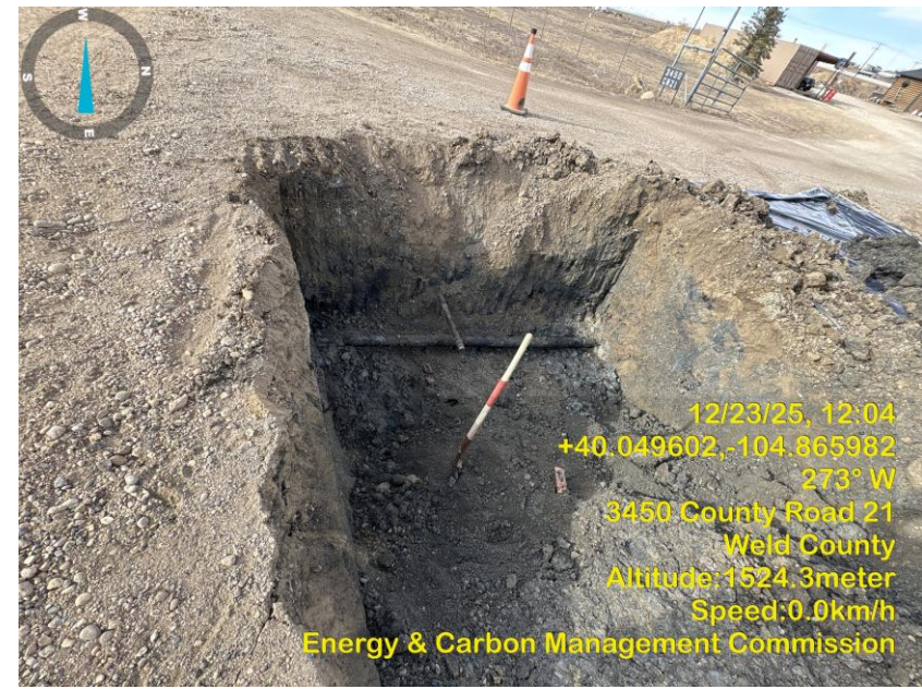
Photo 10 Excavation hole exposing flow lines.
