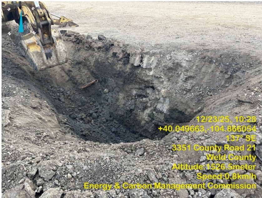
Photo 7 Excavation hole exposing flow lines.
