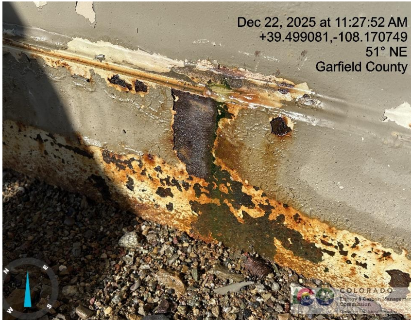
Photo # 4823 Mechanical Condition - Possible separator leak & staining near separator
