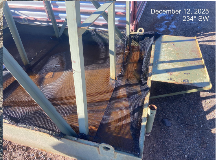
Photo 13. Wildlife protections/coverings at the both the well pads and chem/lube tank secondary containment are insufficient/no longer functioning and need maintenance/replacing.
