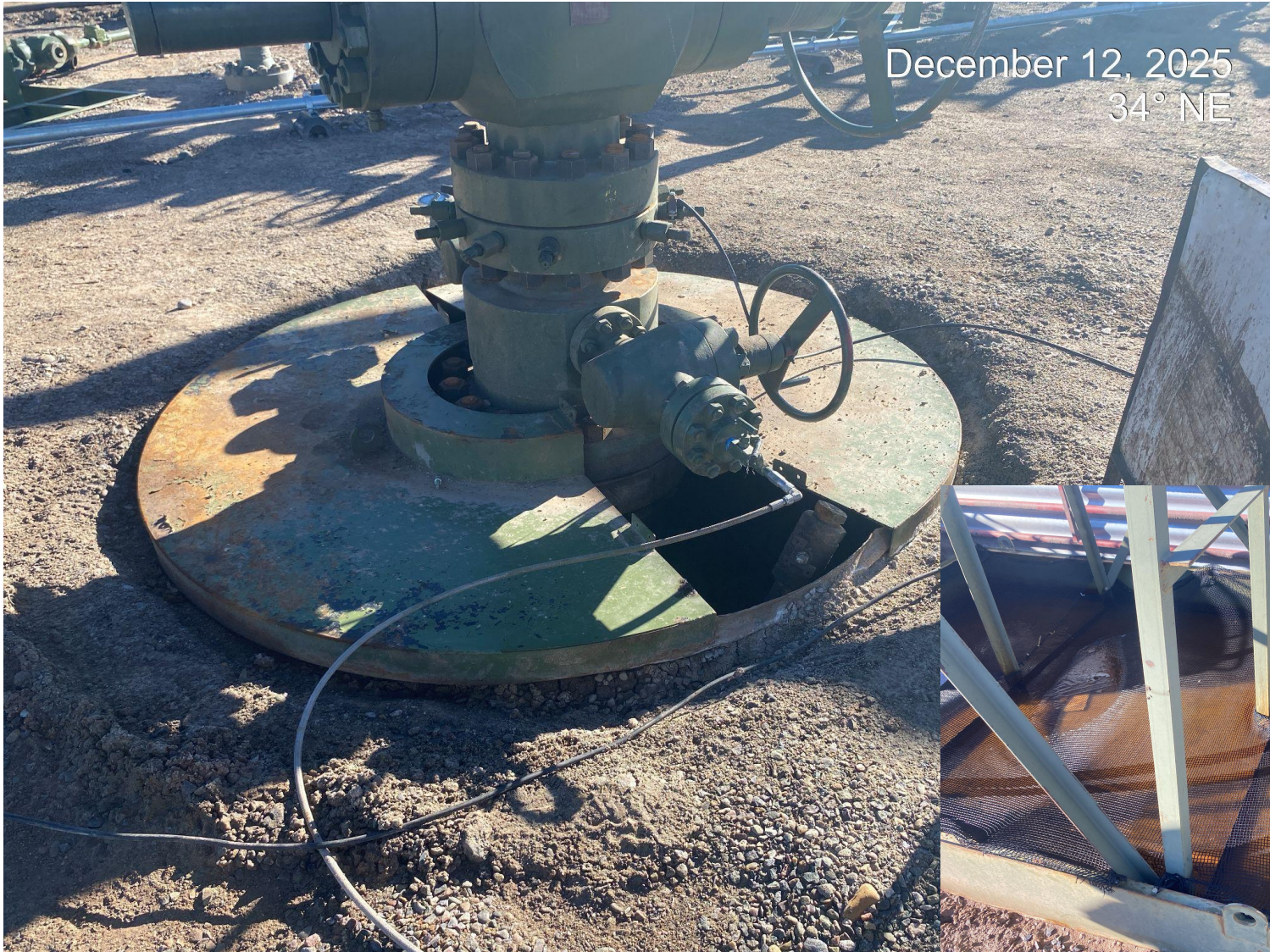
Photo 13. Wildlife protections/coverings at the both the well pads and chem/lube tank secondary containment are insufficient/no longer functioning and need maintenance/replacing.
