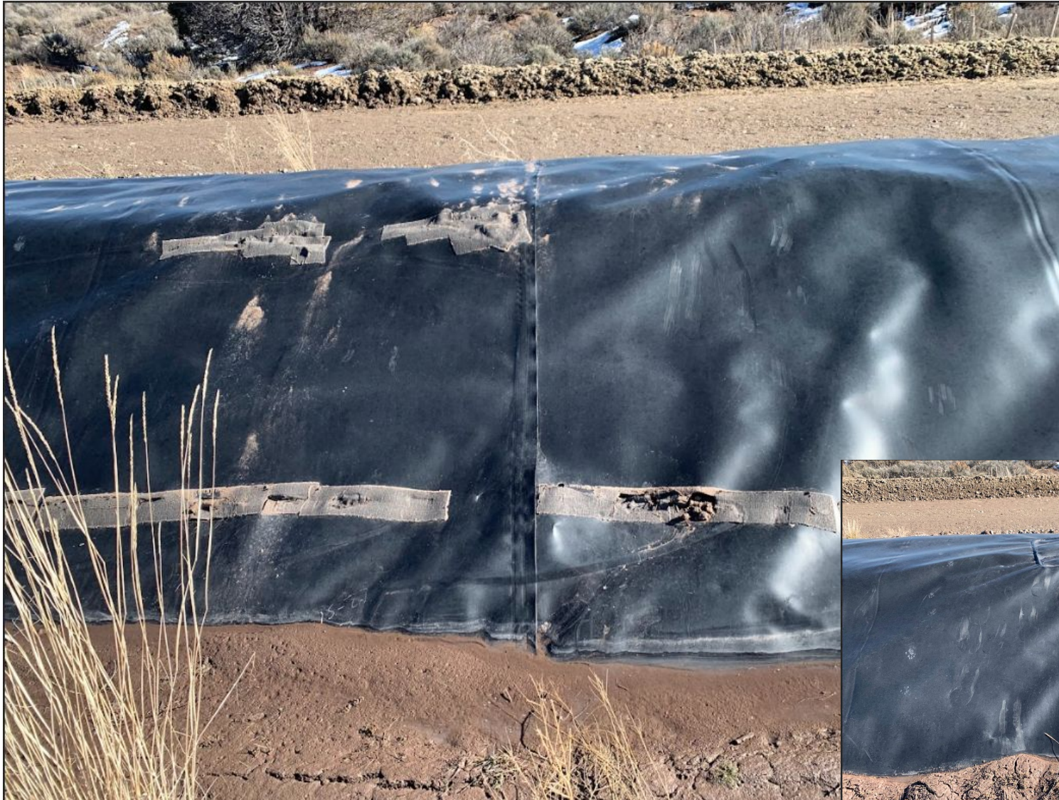
Photo 6. Holes/punctures observed on TUA perimeter berm liner. Existing patch jobs were not successful and holes persist.
