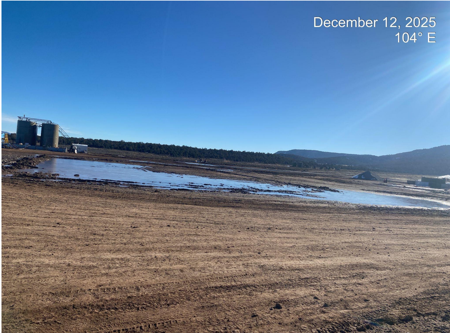
Photo 10. Pooling water observed on the well pad.
