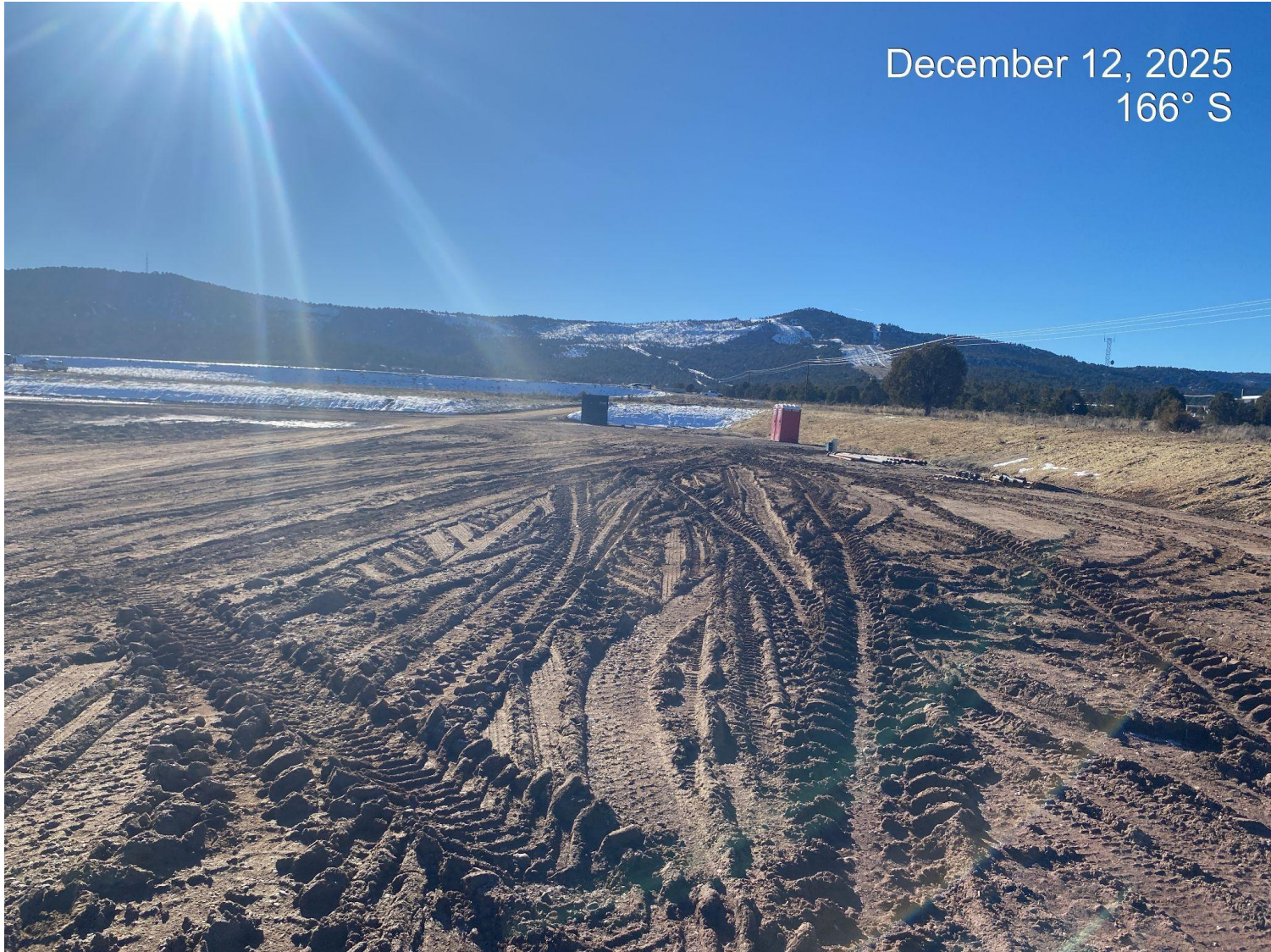
Photo 11. Vehicle tracking observed on the western edge of the well pad. Tracking is consistent with tracking observed throughout the well pad.
