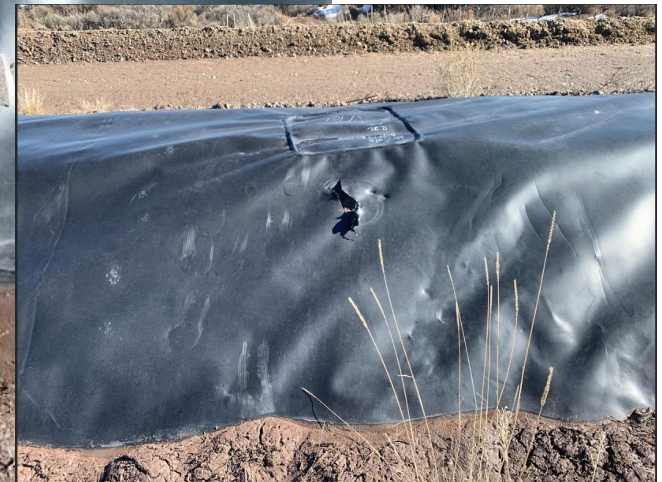
Photo 6. Holes/punctures observed on TUA perimeter berm liner. Existing patch jobs were not successful and holes persist.
