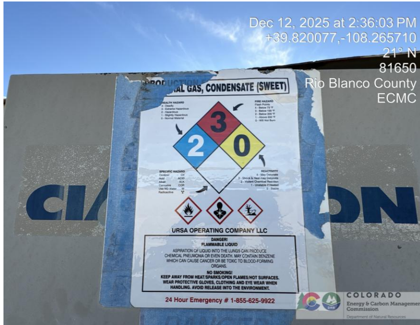
Photo # 0036 Separator door label contains incorrect operator name and disconnected emergency contact number
