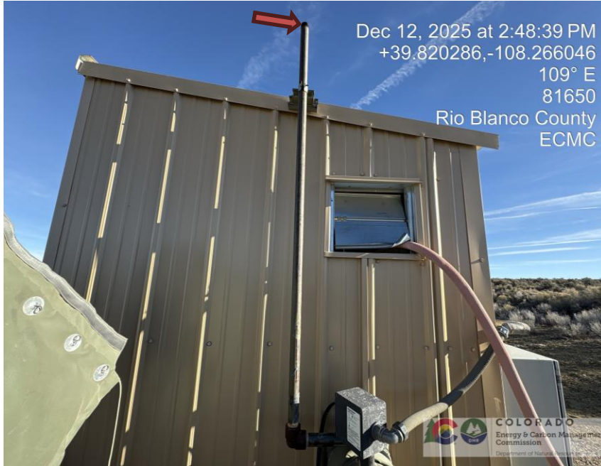
Photo # 0066 PRV vent line does not comply with CECMC pressure safety device rules
