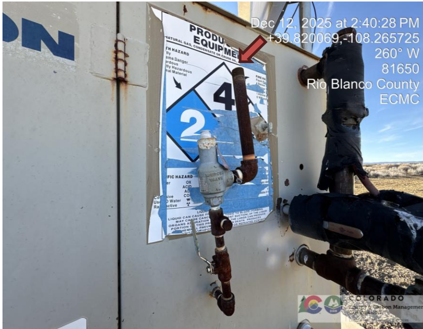
Photo # 0046 PRV vent line does not comply with CECMC pressure safety device rules
