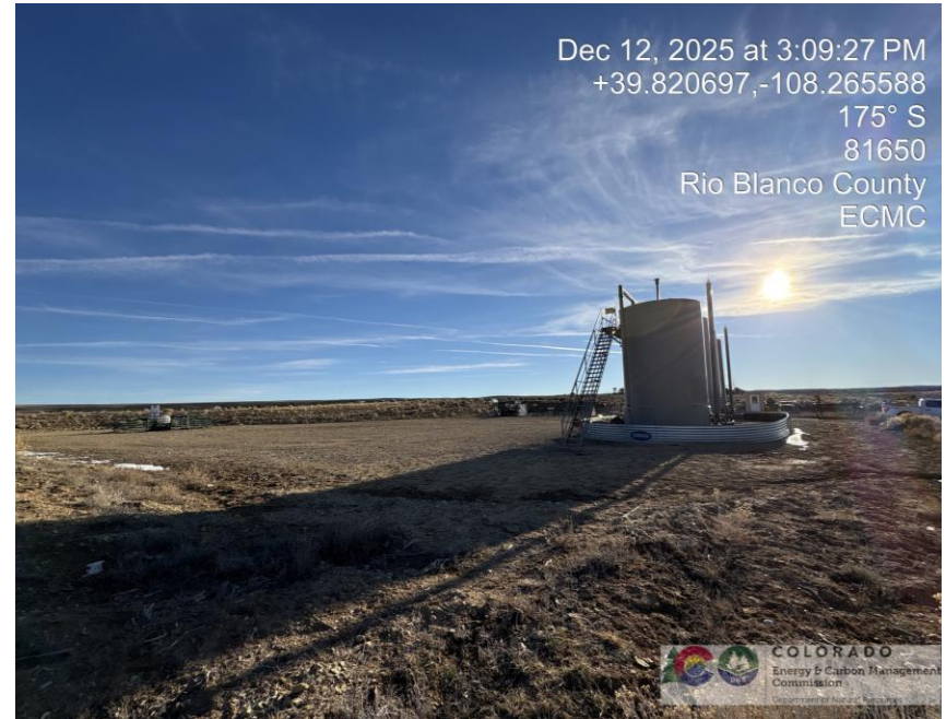
Photo # 0089 NW corner of location
