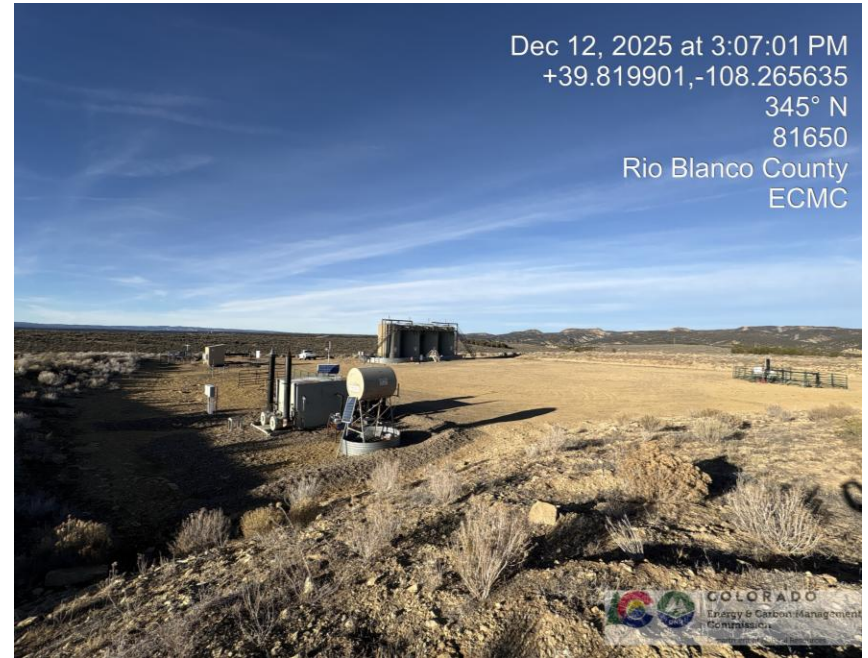
Photo # 0087 SE corner of location
