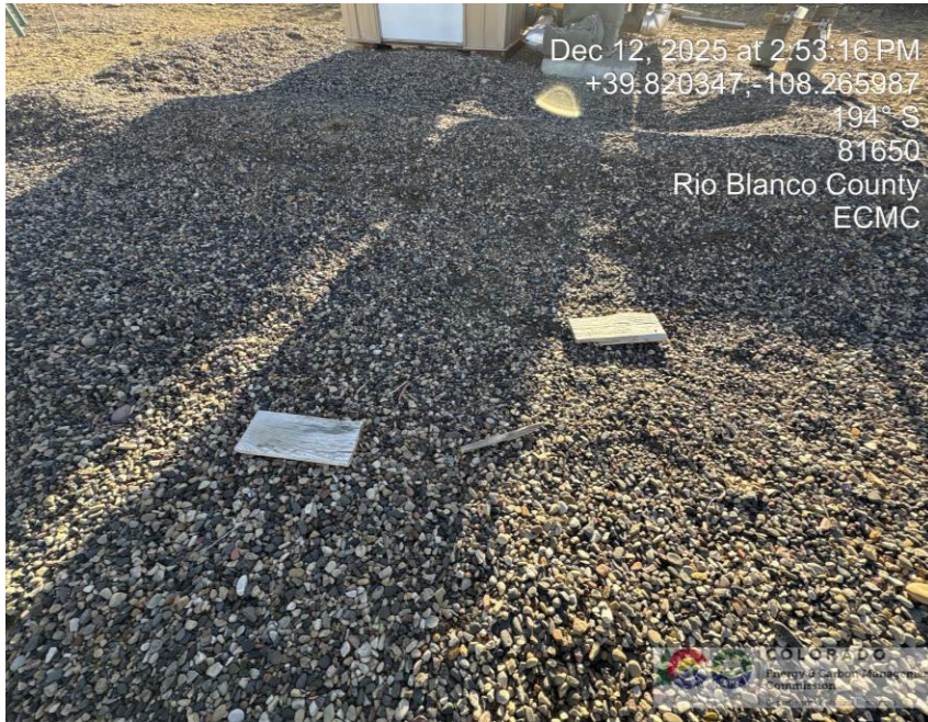
Photo # 0070 Debris on location
