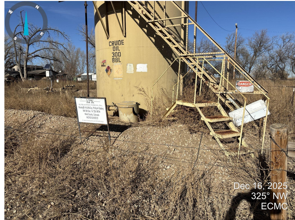
Photo 2. Storage tank and signage.
