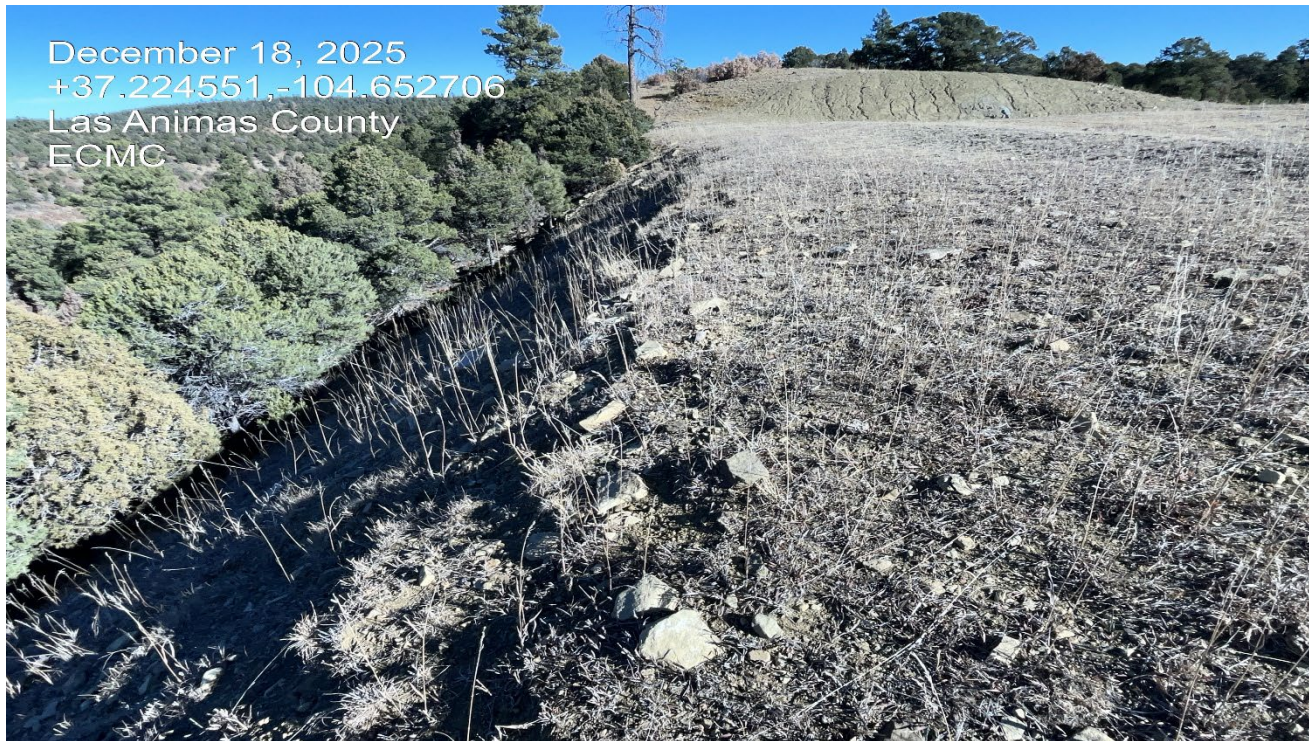
Photo 3. Facing north along the west fill slope.
