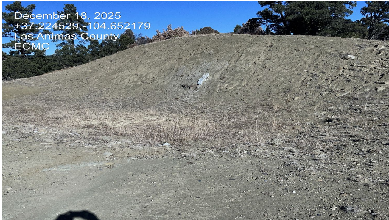
Photo 4. Facing toward the pit that remains. The slope of the pit is not vegetation and there are signs of erosion.
