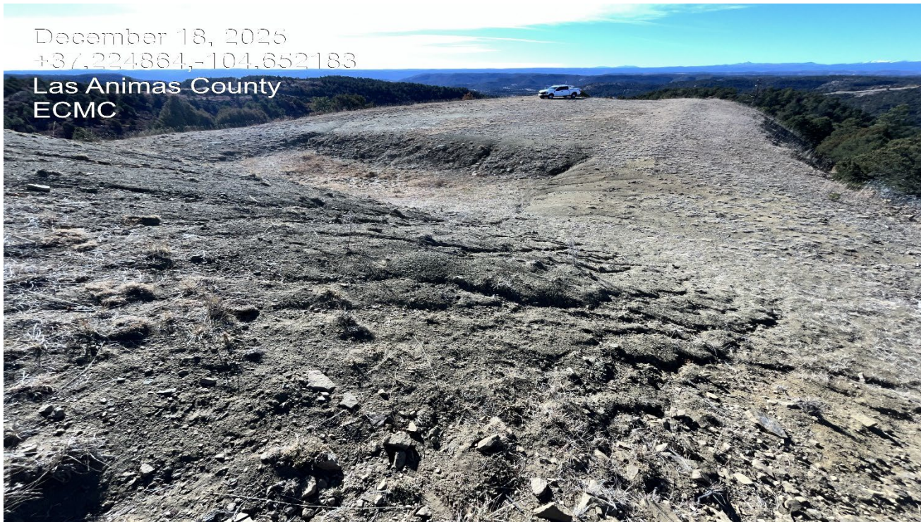
Photo 6. Facing south at the northwest side of the location. There are signs of erosion along this slope.
