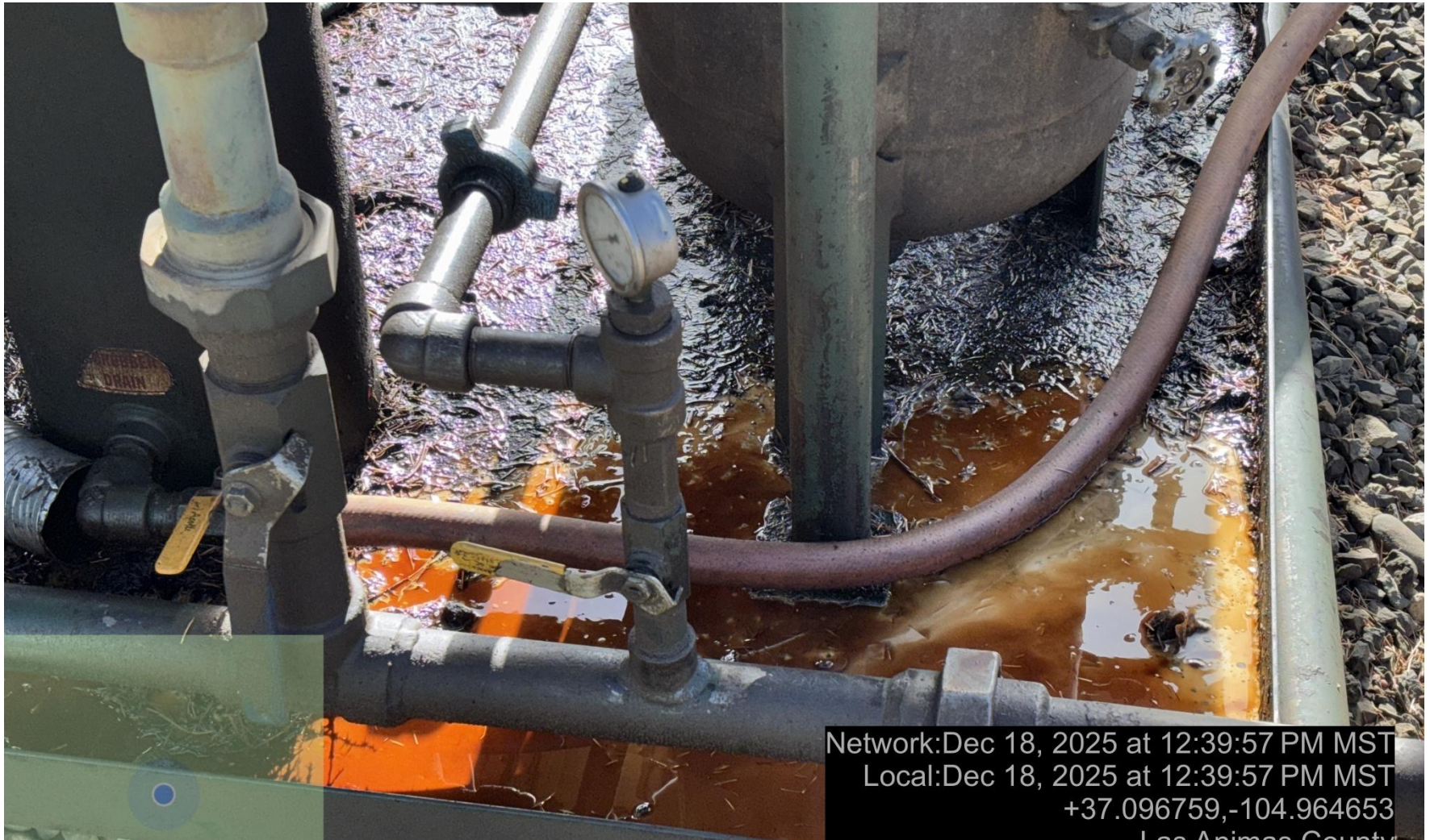
PHOTO 6: OILY WASTE IN COMPRESSOR SKID WITHOUT WILDLIFE PROTECTION SCREENS OR COVERS. DRAIN OILY WASTE REPAIR ALL LEAKS AND REMOVE IMPACTED SOIL PER RULE 1002..(2).D & 1002.f.(2)B, Comply with general provisions of the oil and gas act for wildlife protection AND SB-181. CA DATE 12-19-2025.
