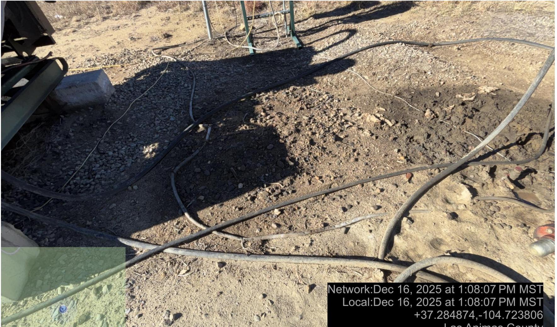
PHOTO 6: AREA OF IMPACTED SOIL BETWEEN WELLHEAD AND PRIME MOVER. Conduct maintenance on equipment, cleanup stained material and review self inspection processes. COMPLY WITH RULE 1002,(2).D. CA DATE 12-22-2025.
